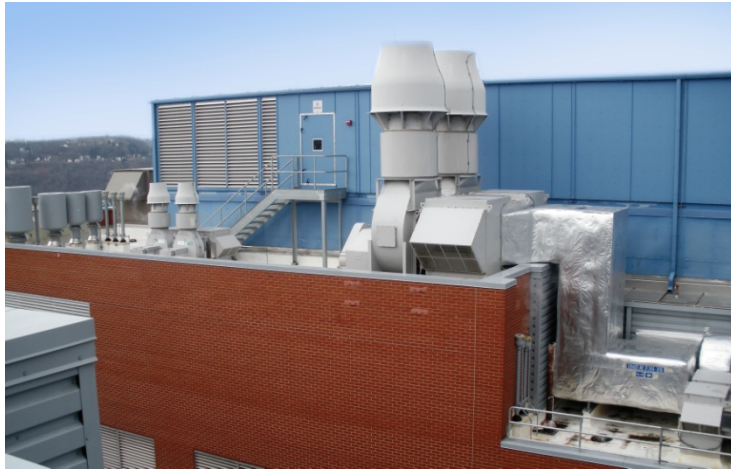
“VariPlume” AMCA 260 Certified Induced Draft Fan (Photo Courtesy of Loren Cook)
