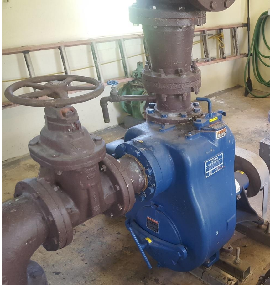
Figure 14: A self-priming, solids handling centrifugal pump, which has a maximum lift height of around 20 feet. Note that these pumps are less efficient than typical end suction centrifugal pumps.
