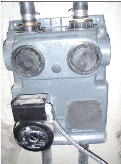
Grundfos Flow Controller Model AFCG2C1 With earth loop pipes above and heat pump rubber pipes below, as installed. Approximate purchase cost is $700.
