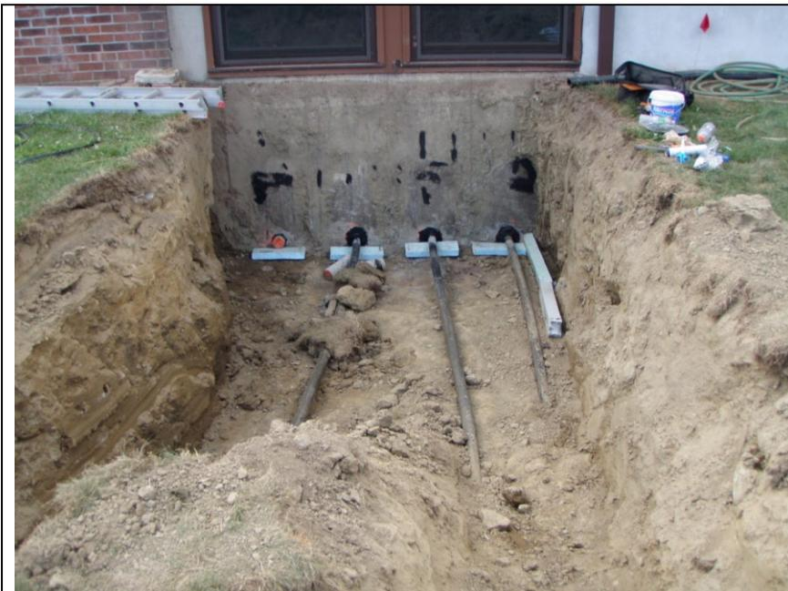
**Figure 30 Inlet and outlet loop insertions into basement.**
