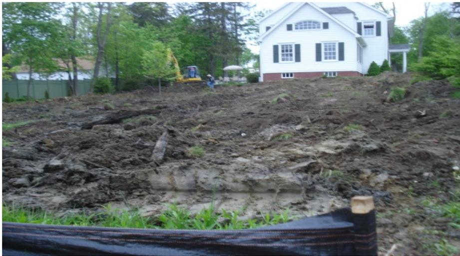
**Figure 8 Silt fence erosion control.**
