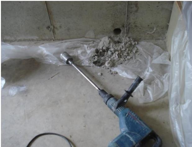
Figure 27 Dry drilling that creates concrete dust.
