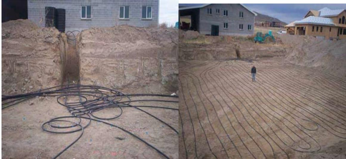
Figure 16 Complete dirt removal versus trenching. (<http://www.geoexchange.org/>)
