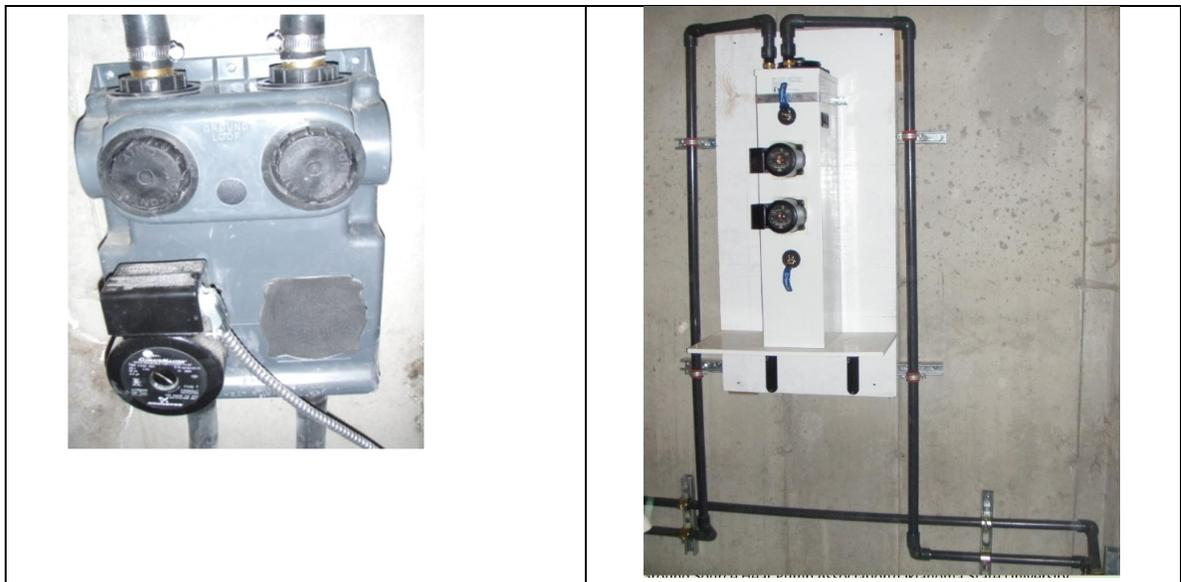
**Figure 19 Grundfos Flow Controller Model AFCG2C1 with earth loop pipes above and heat pipe rubber pipes below. Approximate purchase cost is \$700. Non pressurized flow center option, to the right. It is actually about 5 psi and available with smart controls. They can be more costly, but could eliminate the need for flushing.**
