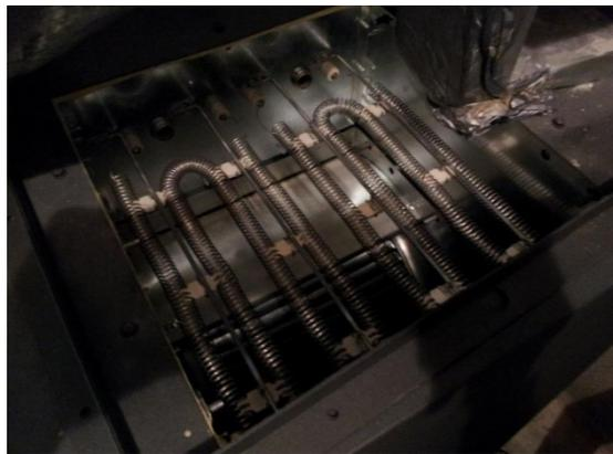
***Figure 15 Inefficient (COP=1) Duct Heater,
