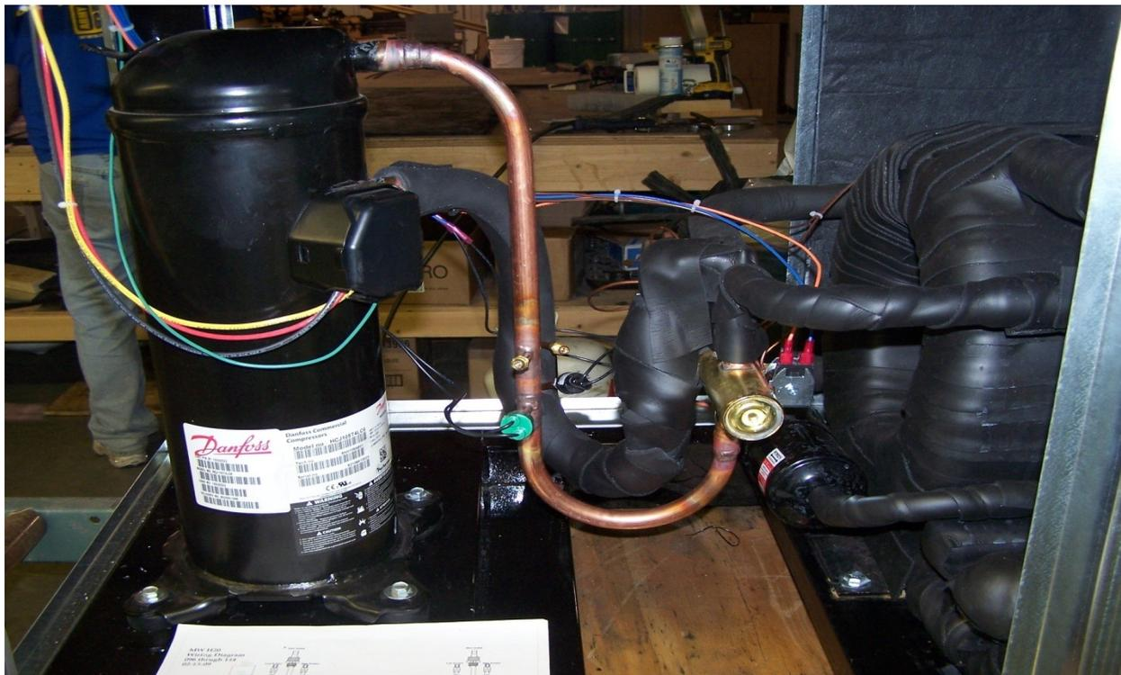
**Figure 6** Copper tube assembly going from brass reversing valve to the condenser coil.
