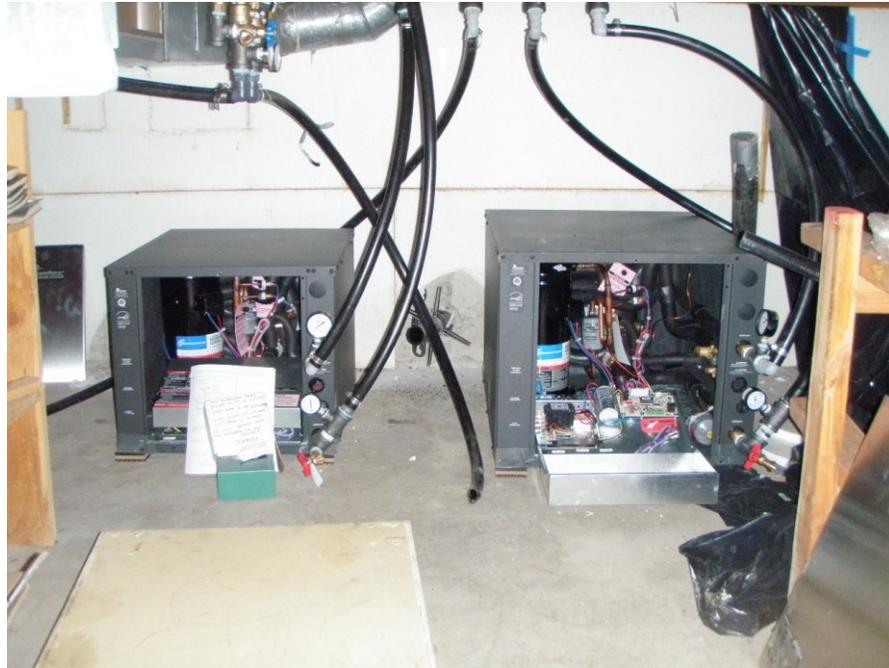
**Figure 16** Two-stage split GSHPs being installed in a crawl space.
