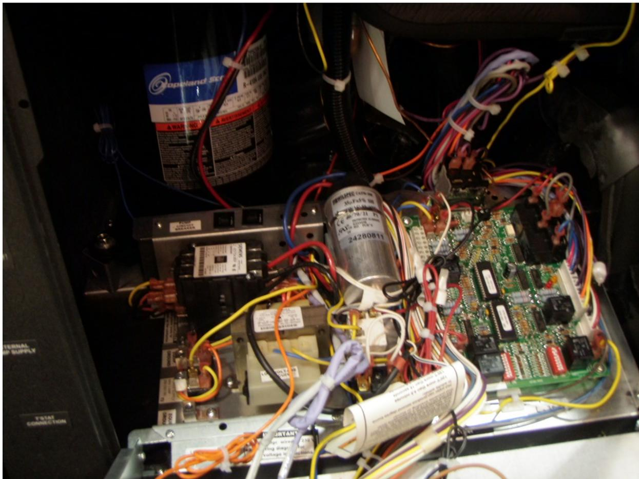
*Figure 23 Control panel circuit board inside the split cabinet of a GSHP next to the compressor.*
