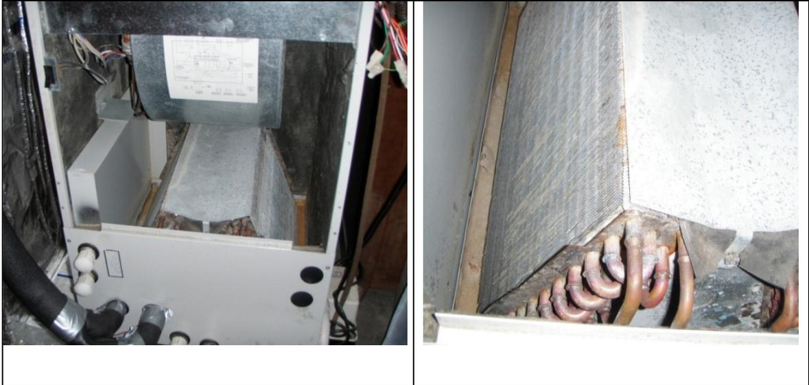
*Figure 8 Condenser detail within the air handler cabinet. Copper tubes circulate R-22 here. (In the field, the technician will call this the evaporator coil, referring to its use in cooling mode.)*
