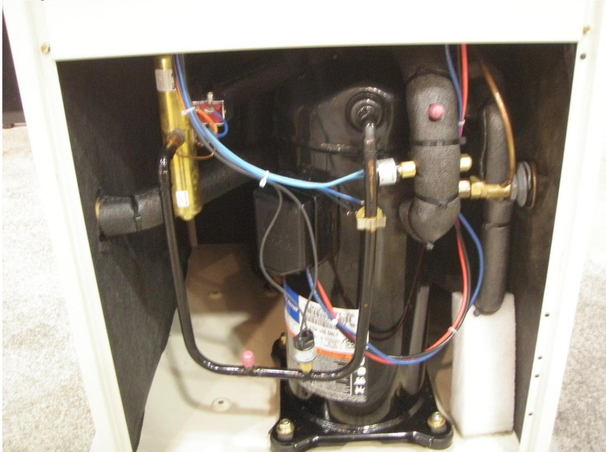
*Figure 4 Interior components of a Copeland dual stage compressor (compare to two gears in a car).*
