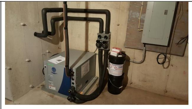
*Figure 34 Split System installed close to wall loop penetration with flow center & 10 gals of antifreeze.*
