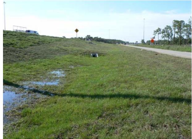
**Figure 17: Ground Drops Away from Culvert Outlet**
