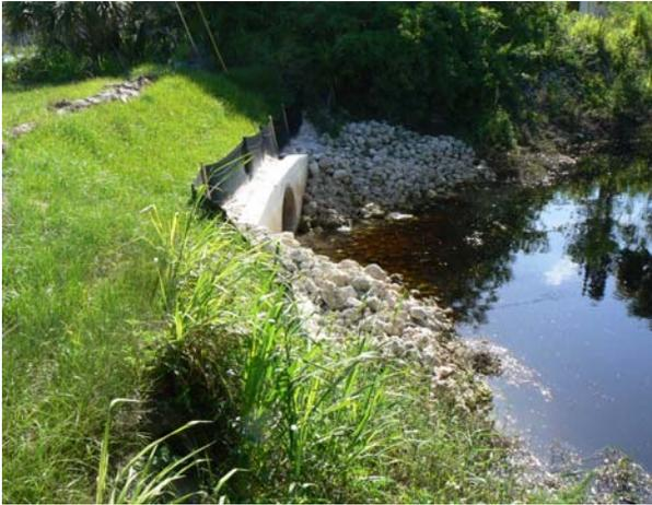
**Figure 16: Pond Outfall into Existing Stream/Lateral Ditch**
