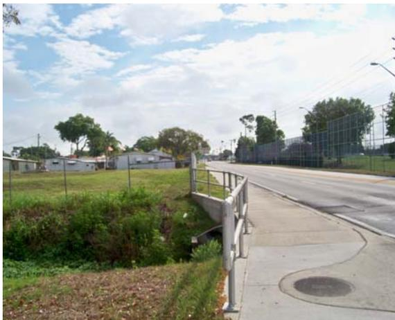
Figure 10: Cross Drain Outlet
