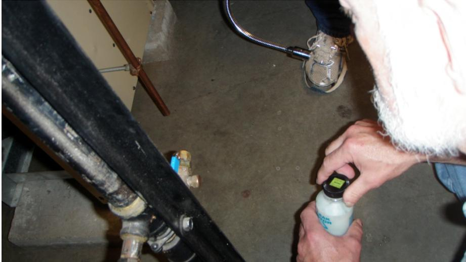
*Bubble detection for Gas Leak*
