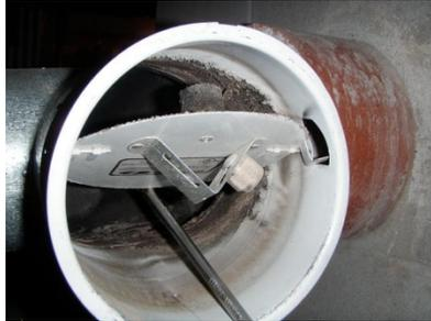
*Damper flap. Test both pressure and CO level.*
