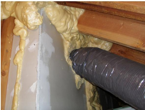
*Foam air sealant around duct opening*
