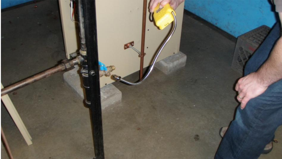
*Proper gas leak detection.*
