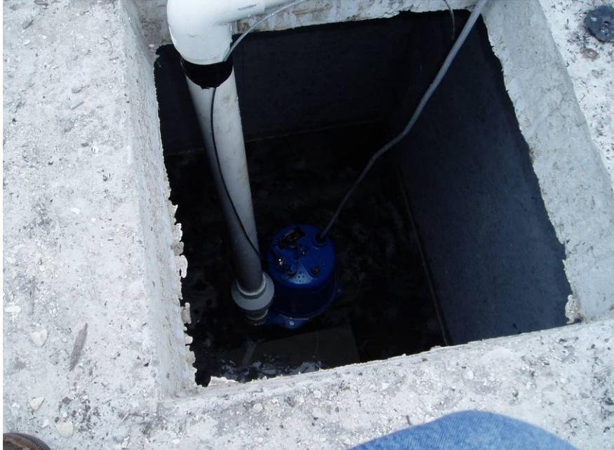
A septic dosing pump installed in a tank
