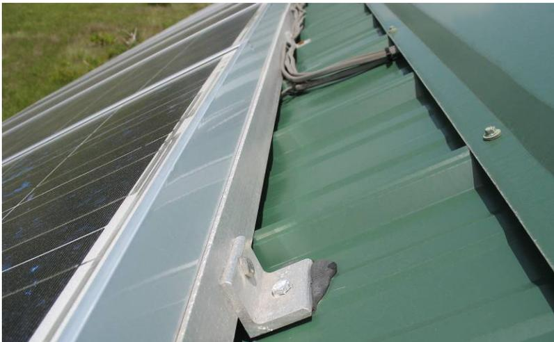
Notice that no conduits are used for the panel wiring. This should be noted and then corrected by the installer.
