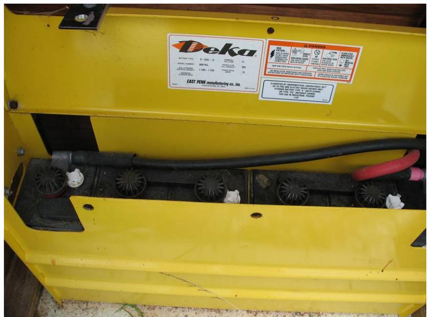
Another check is determining if the batteries maintain a charge overnight with no loads on them. If the voltage decreases overnight with no load, the batteries will need to be replaced.
