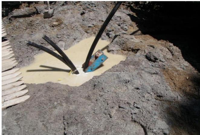
2. Then the grout colored water flows out, as the entire borehole is filled solid with only the two 1 1/4" loop pipes, and the grout.
