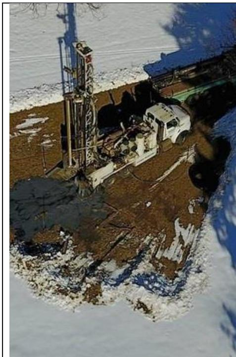
The GeoCube thermal conductivity / thermal response test unit and the associated boot camp training prepare the user to perform a thermal conductivity test of a borehole. The author recommends this one day course after taking it himself. For pure electric power sources, the software plots temperature against time and uses the graphed slope to determine thermal conductivity of the formation below. Geothermal Training Institute in Maple Plains, MN offers occasional training.
