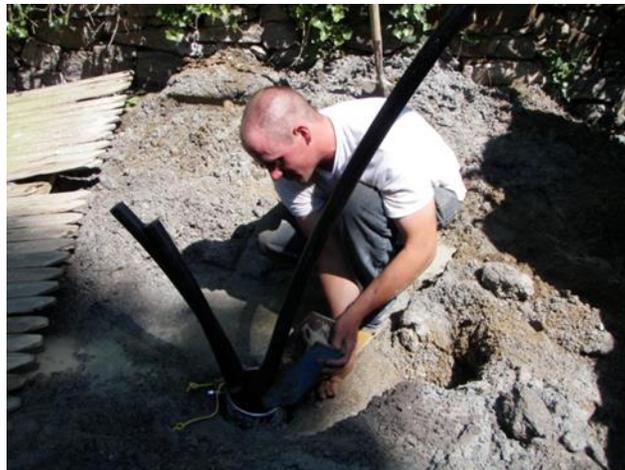
**Figure 21 Twin rollers attached to the casing make insertion easier.**
