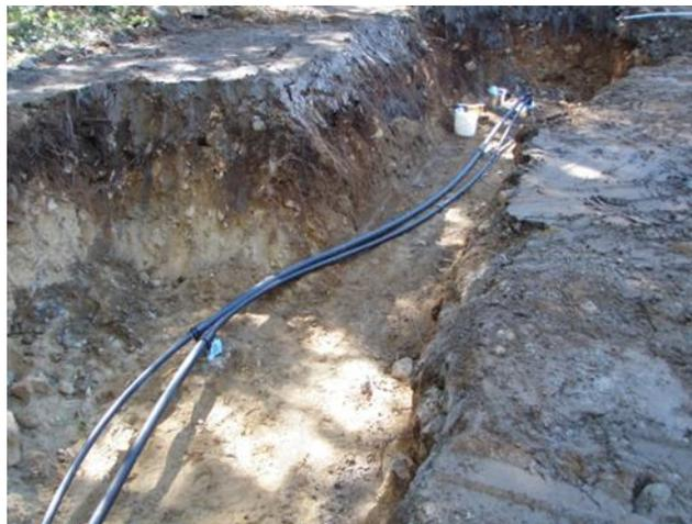
6. The Horizontal Reverse Return with 2" and 1 1/4" HDPE connects the boreholes to the building. It is now ready for backfilling.
