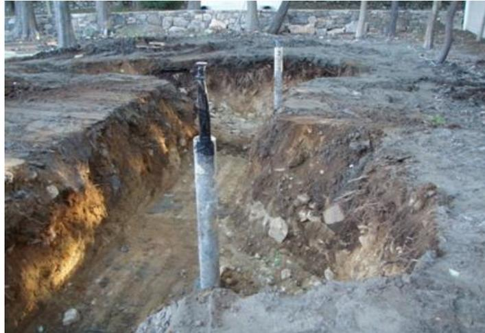
3. After the grout sets, an excavator digs a 4' to 5' deep trench to the building and the steel casing in ledge, will be burned off 4'-5' below the surface.
