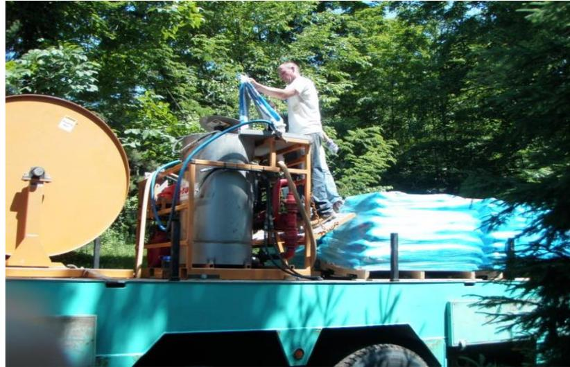
**Figure 24** Adding silica sand and bentonite grout.
