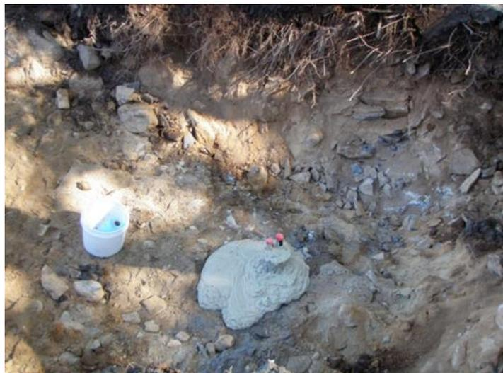
4. Bentonite grout is not set even days later, like cement grout. It feels like wet, sandy peanut butter. Here it has slumped after the 5' casing was cut.
