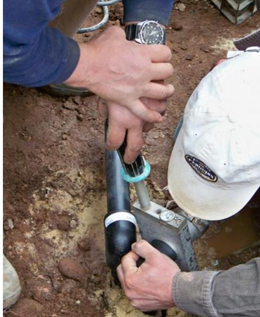
5. 90-degree elbow bends and tees are socket heat fused onto each vertical loop pipe end, to run a horizontal HDPE into the building. Alternatively, the HDPE can be carefully bent 90 degrees and butt fused horizontally.
