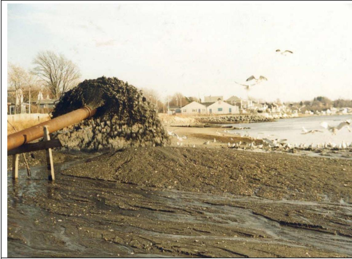
Figure 1: Gravelly sand being placed on a beach as part of a nourishment project.
