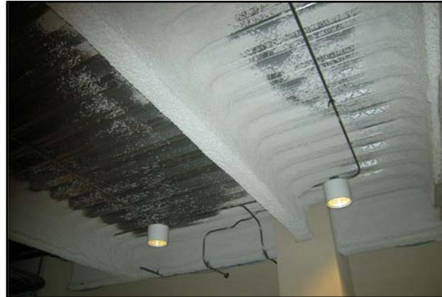
Photo No. 13 - Spray-on fire protection
