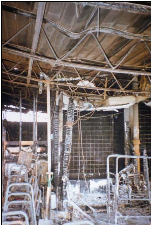
*Photo No. 11 - Steel bar joists after a fire.
