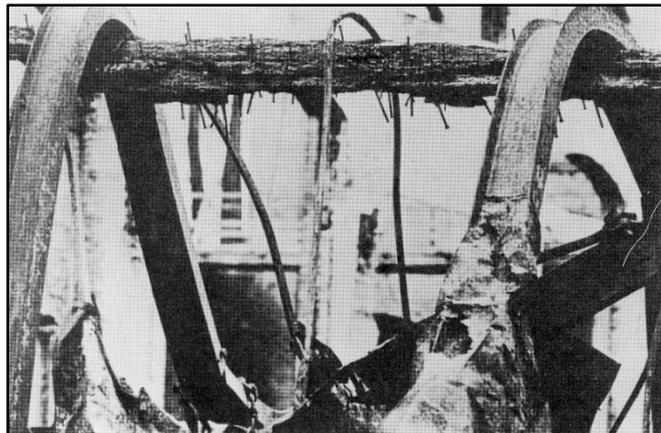
Photo No. 14 - Fire reduced strength of steel to zero
