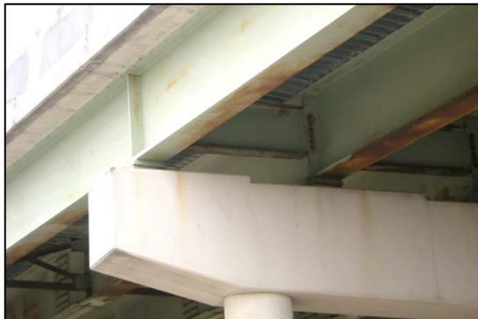
*Photo No. 17 - Stiffener plate at support*
