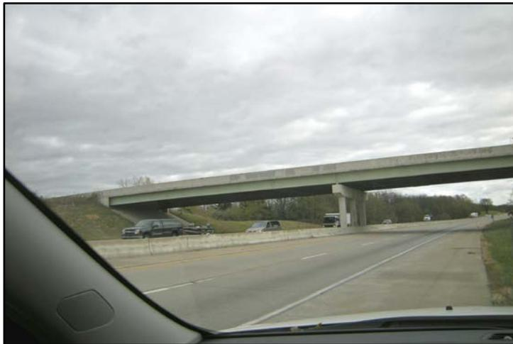
Photo No. 3 - Typical 2 span continuous bridge beam
