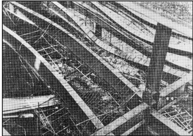
*Photo No. 10 - Steel beams after a fire*
