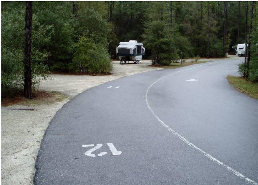
Campsite signage may be handled in multiple ways but my preference for campgrounds with paved drives is for the numbers to be painted on the asphalt in 12-inch letters with reflective paint. The painted numbers are easy to read day or night and are also easily maintained. The numbers should be painted either in the center of the campsite driveway or adjacent to the drive's edge of pavement.
