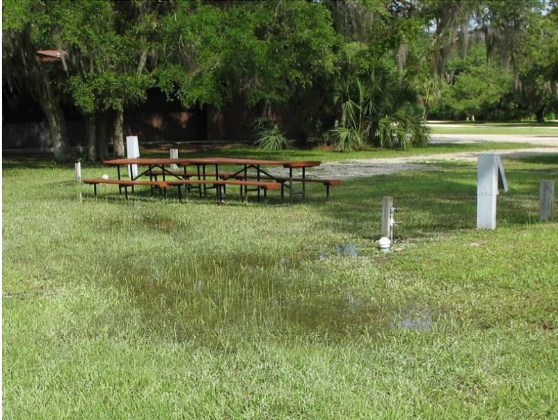
*Poor drainage at campsite - notice utility services are located in standing water*
