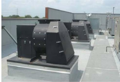
*Upblast Centrifugal and Upblast Ventset (with EasyClean coating) Exhaust Fan Styles
