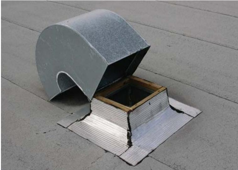
A seemingly simple installation of a “gooseneck” duct termination can be problematic in a wind and rain storm. It isn’t just the damage to the roof and equipment that is of concern, it also becomes a more serious concern when water can enter a duct system and distribute in a building causing extensive water damage throughout the building.
