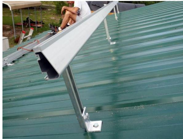
*XRS rails with upper and lower mount brackets installed. The end caps must be installed after the solar panels are attached.*
