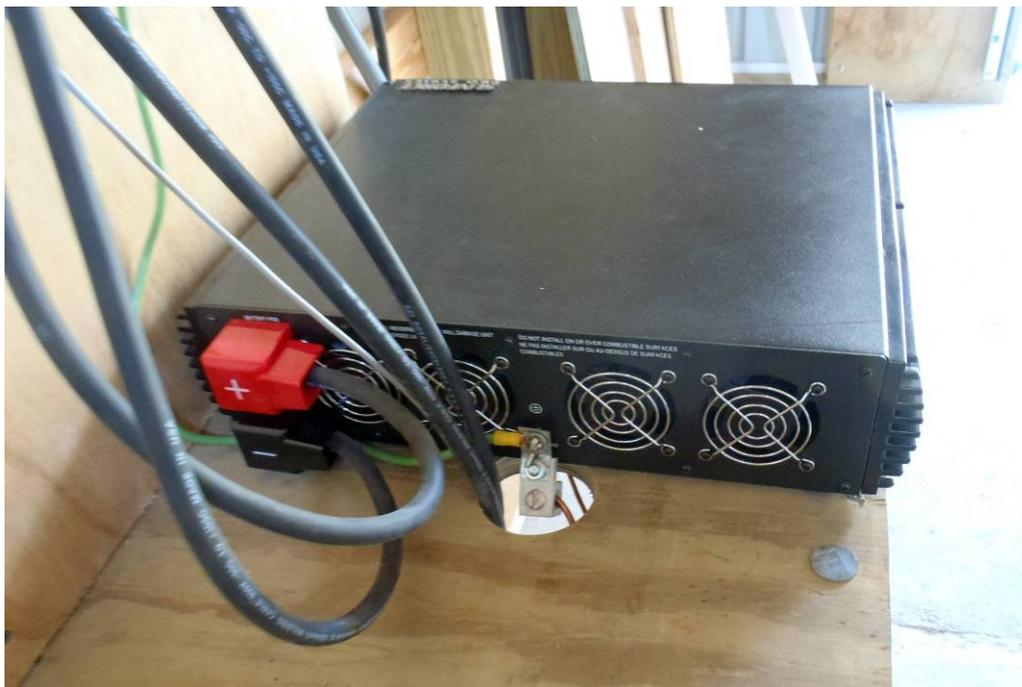
*DC Connections in the rear of the SunForce Inverter*
