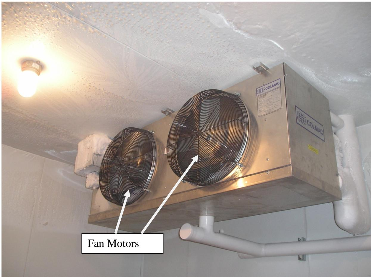
Arriving at the correct fan power value is an iterative process, as the total space load must be determined in order to select the evaporators, then the fan power must be adjusted to match. A good starting point is to estimate 0.25 HP/Ton.
