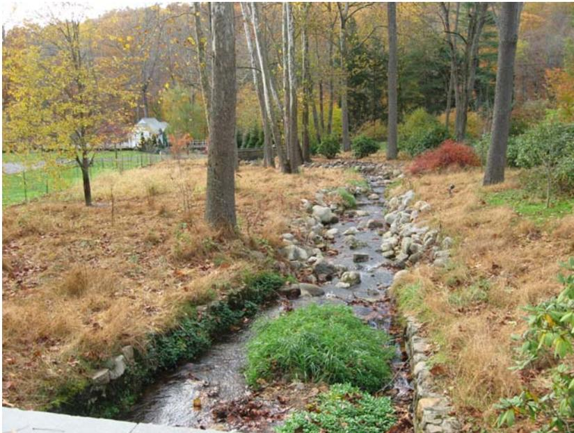
The three main design parameters vegetated for filter strips are its slope, vegetation type, and its soils. The maximum filter strip slope can be determined from the table below:
