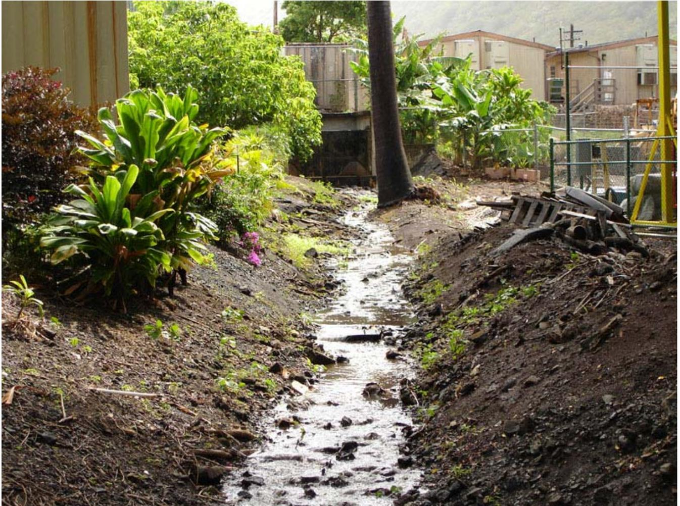
Based on the facts presented in this course, however, it is apparent that this swale is not very efficient in treating the runoff. The photograph shows a fairly straight, somewhat poorly-vegetated swale flowing through an urban area. Several things could be done to increase its filtering capabilities. These include the following:
