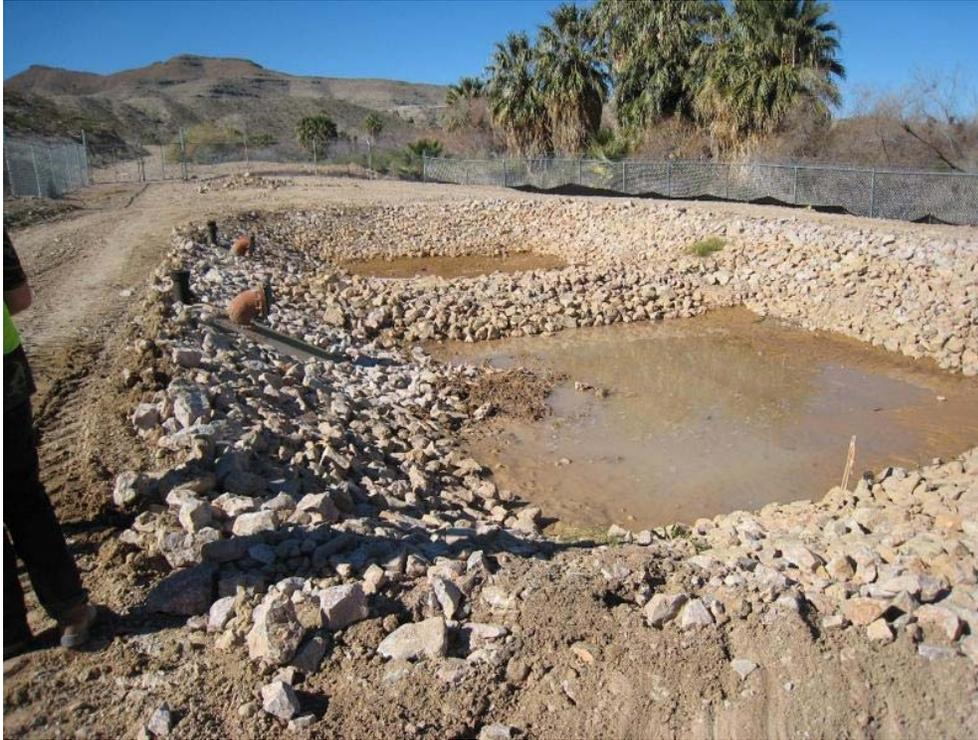
The photograph at the left shows an infiltration basin in an arid climate. This photograph was taken from the Nevada Division of Environmental Protection website.
