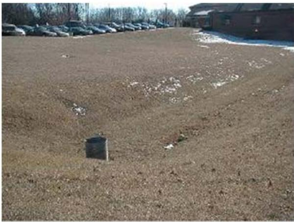
The photograph shown at the left, taken from the USEPA website, shows a typical infiltration basin. An overflow box is shown in the foreground.
