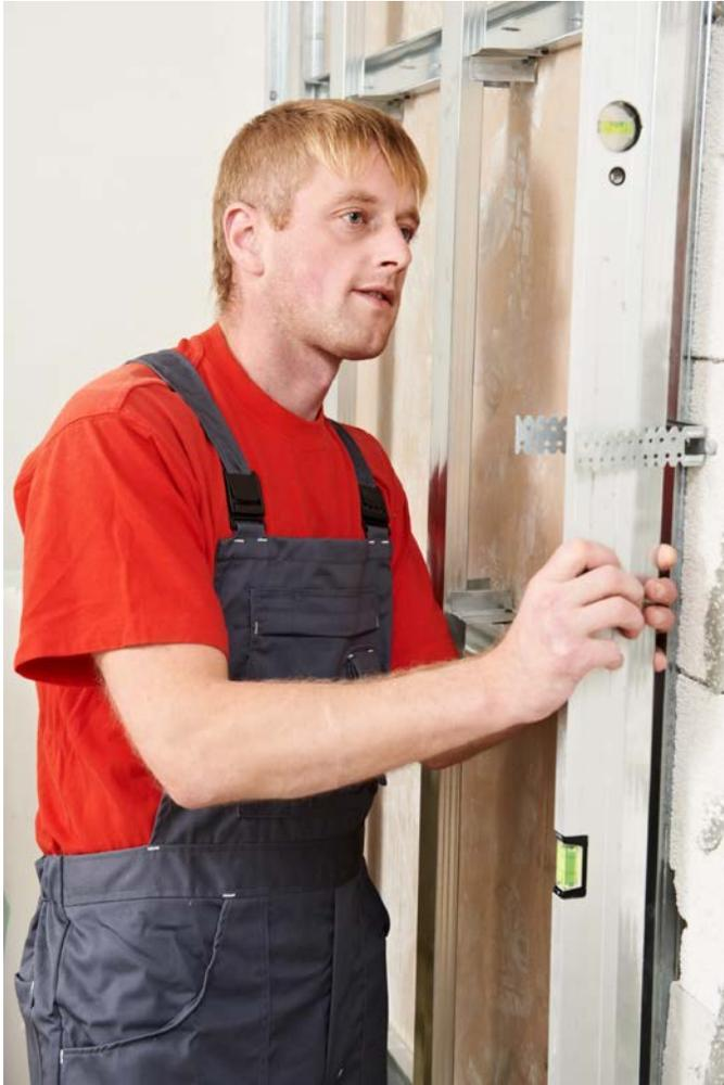
Picture No. 5 by [www.canstockphoto.com](http://www.canstockphoto.com) Interior partitions, where wallboards are usually installed on both sides. All wallboards, including Sheetrock and Drywall, are asbestos suspect materials.
