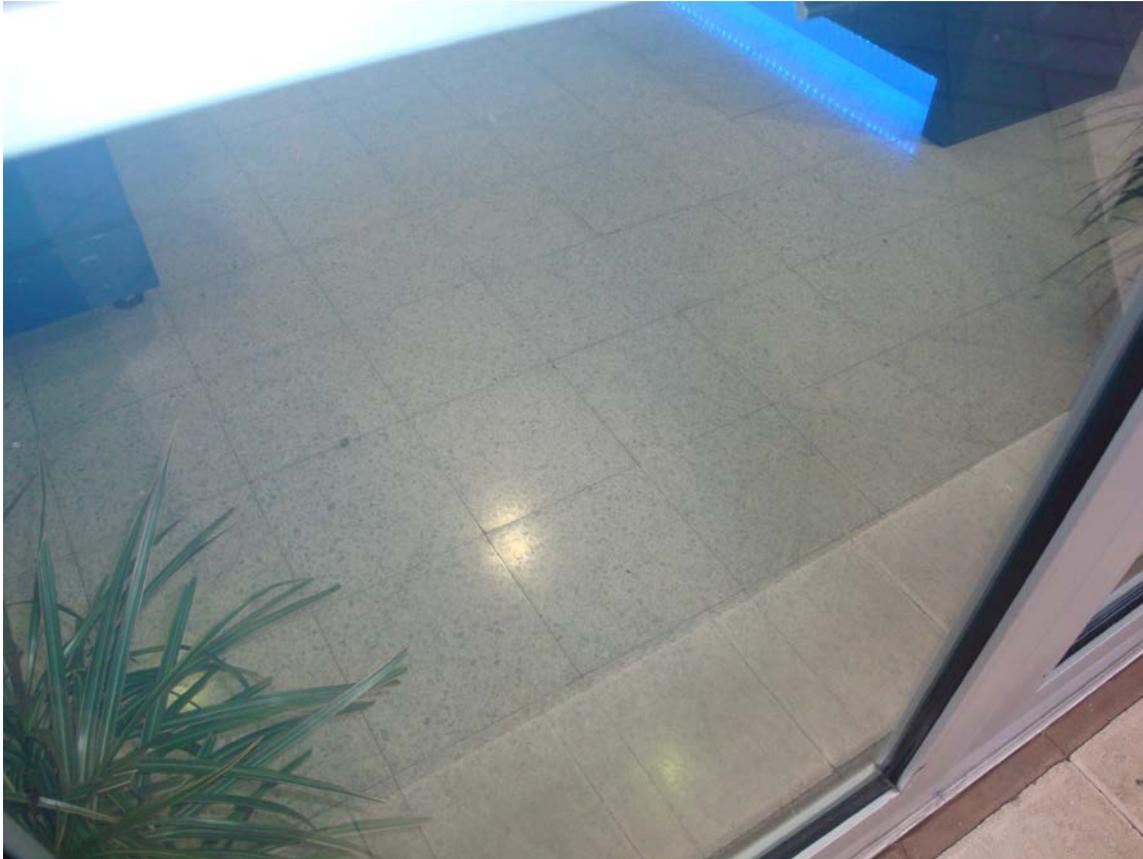
Picture No. 4 by Author. Vinyl Floor Tile, size 12" X 12". All Vinyl Floor Tiles (VFT) including sheeting are also called Resilient Flooring and are asbestos suspect materials. The 9" X 9" Tiles are highly suspicious of being ACM
