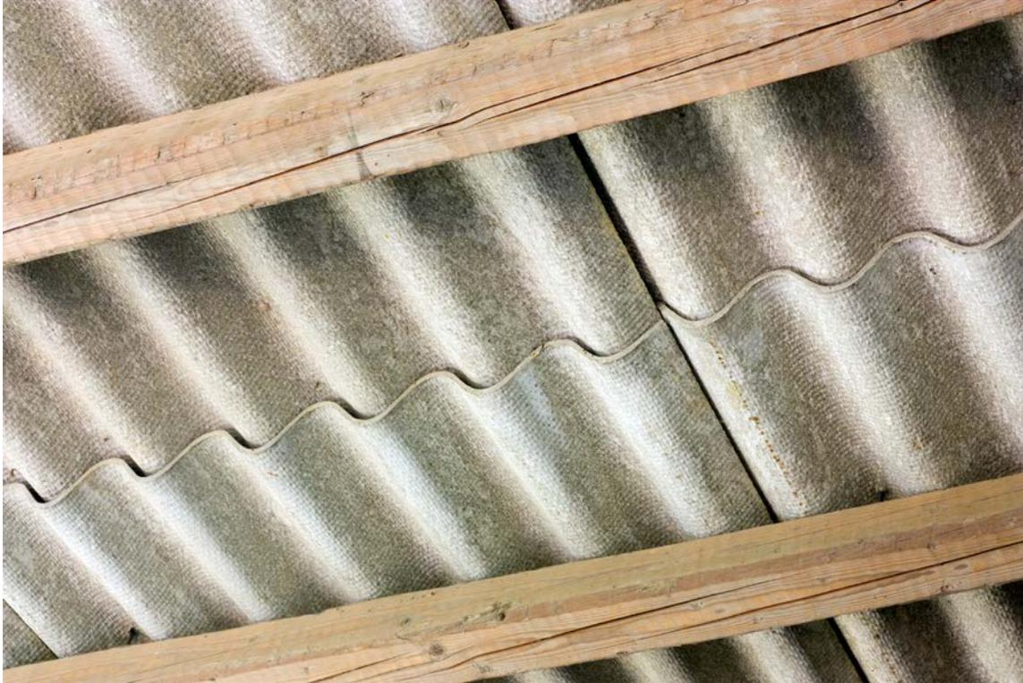
Picture No. 3 by [www.canstockphoto.com](http://www.canstockphoto.com) Corrugated Cementitious Roofing Boards or Transite Boards. They are found all over the world, and can be quite dangerous if disturbed
