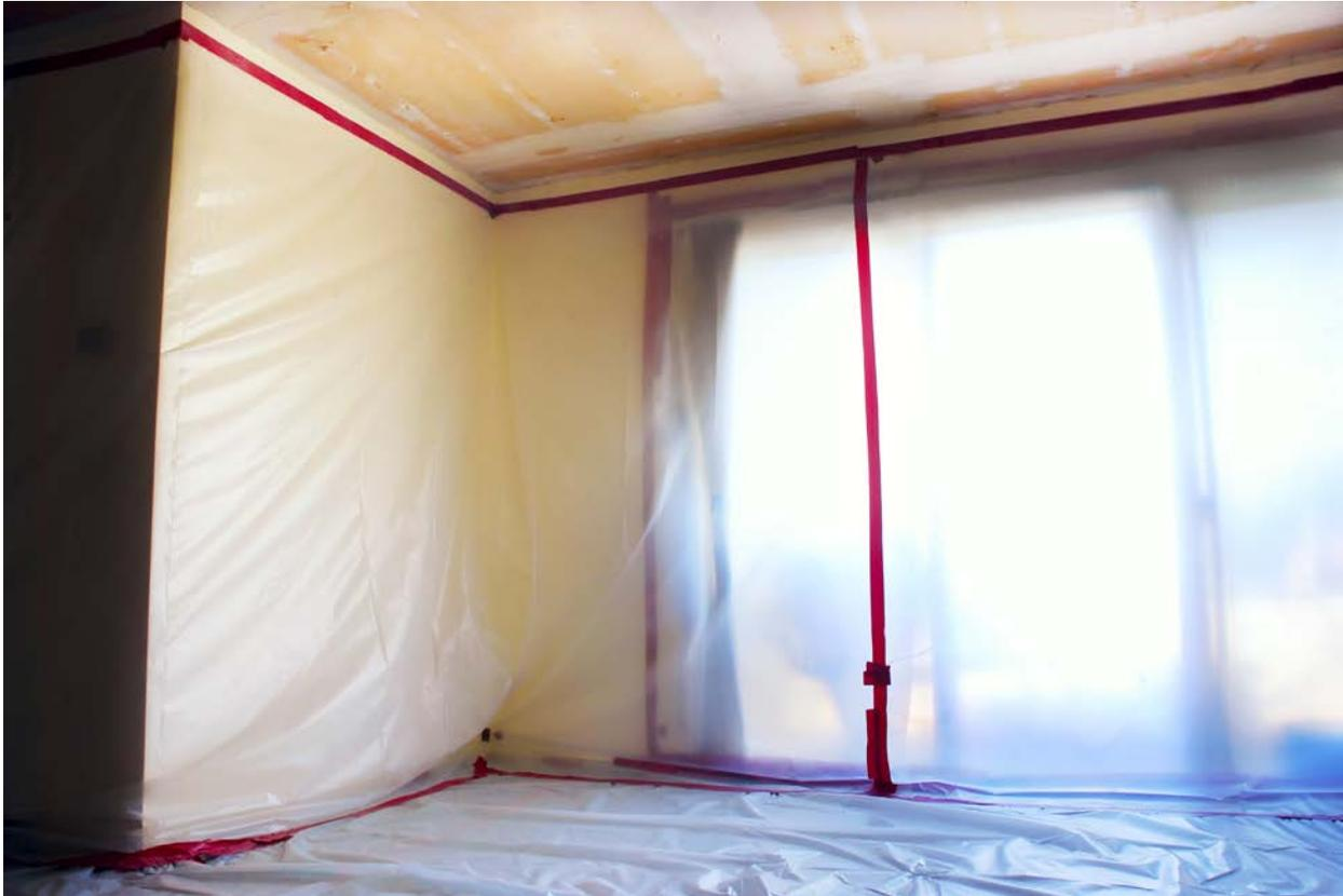
Picture No. 6 by www.canstockphoto.com NPE with the polyethylene sheeting in place. Popcorn ceiling or similar coating appears to have already been abated.
