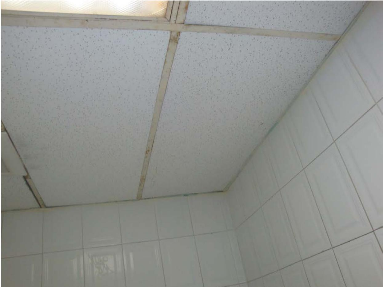
Picture No. 10 by Author. Acoustic or ceiling tiles having minor water intrusion damage. The regular surveillance activity should pay particular attention to materials where decay or damage has already started. Friable ACM Tiles such as these are still legal to install in the US
