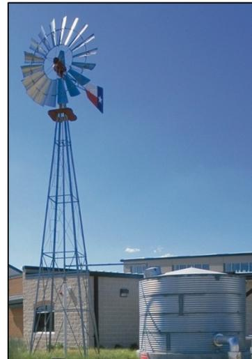
**Figure 1 - This windmill with fantail in Texas is an example of an HAWT. Photo by Scott Milder, NREL 10678**
