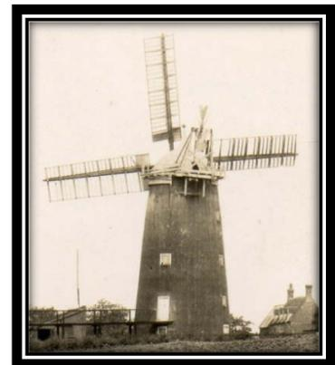
**Figure 3 - The blades of a Dutch-style windmill rely on drag for moving.**
