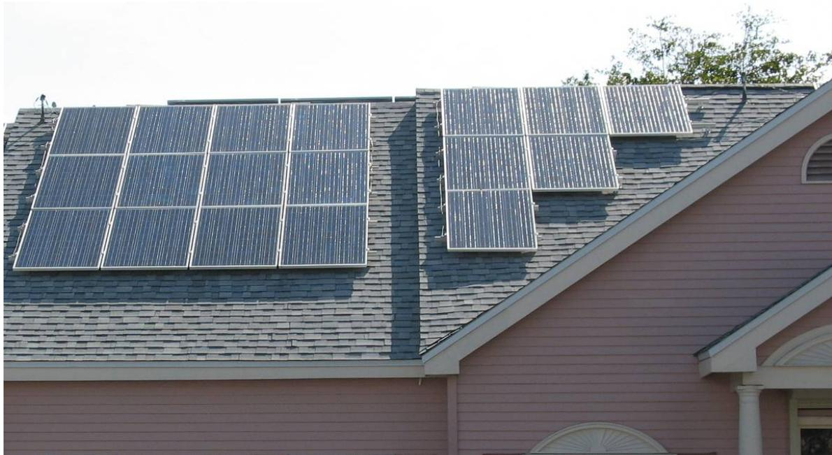
**STC Ratings** – Solar panels are rated under Standard Test Conditions (STC) by the manufacturers at 1000 watts per square meter of solar irradiance at 25° C. If the temperature is different than 25°C (77°F) or the sunlight intensity is different, then your panel will perform differently than the specifications stated. If you have high power demands but have limited space, you'll need to select panels with the highest ratings.
