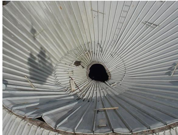
Cause and Origin: this is one of two 90-ft diameter grain storage silos out of four at the same site. The steel roof on each failed suddenly inward. There was weather in the vicinity. Was this weather, a construction defect, or could it have been something else?
