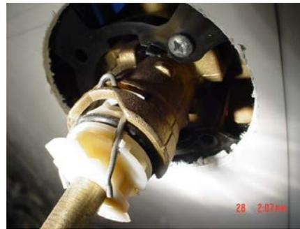
This shower valve cartridge was forced out of the body of the valve by freezing. This occurred because the contractor left the area unheated during freezing weather and this is therefore a construction defect.
