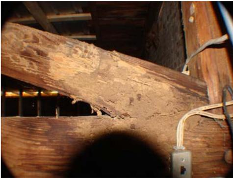
A flat, trussed roof partially failed after a heavy rainstorm. The root cause of the failure was long-term termite infestation, and a secondary cause was the weight of ponded water on the roof.
