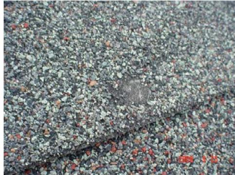
For hail damage cases it is very important to have good macro photos of the indications. Indications should be compared with available photos of typical hail and non-hail damage, and the photo is also very useful to demonstrate granular loss and damage to the mat of the shingle. It is not enough to just state that there is hail damage, you also have to *demonstrate* it.
