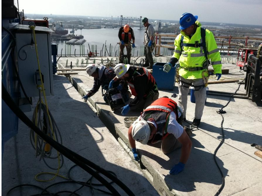
Spreading epoxy lubricant/sealer between segments prior to tensioning
