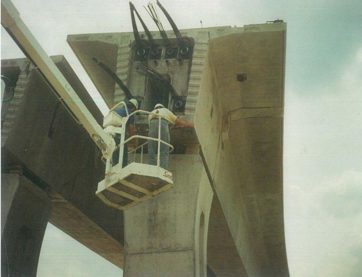
After the setting and joining of the span is complete, the post-tensioning operations will begin. Install permanent internal and external post-tensioning strand and rod longitudinally through the span. The number of strands per duct and the number of ducts per span will vary and a stressing sequence will be provided in order to transfer a uniform load. The strand is stressed using high strength hydraulic jacks. When the
