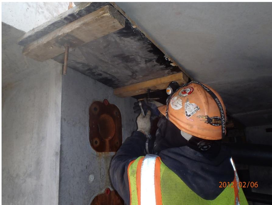
Forming span closure pours from interior of segment box
