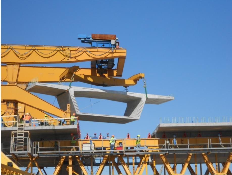
Gantries lifting segments using under wing straps with softeners at the concrete edges
