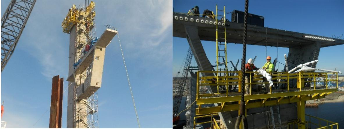
**Strongbacks:** Any segments requiring a closure pour that cannot be supported from below using shoring towers will need to be hung in place using strongbacks until the closure pour concrete is hardened and the post-tensioning steel is stressed. Strongbacks are steel beams which are anchored to the previously erected superstructure elements and hold the subsequent segment in a cantilevered position.
