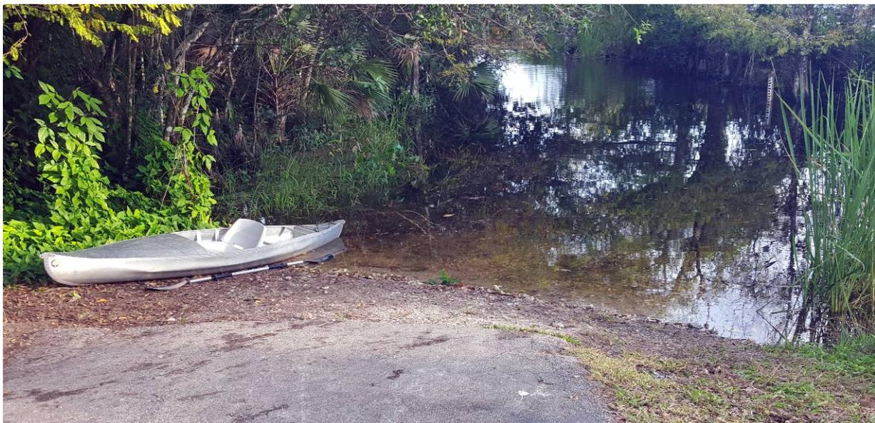
*An asphalt paved ramp to a natural shore line for launching*
