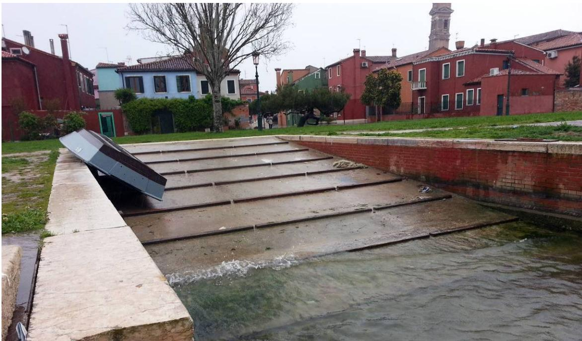
*Figure 18 – A concrete NMB ramp with wood runners in Burano, Italy*
