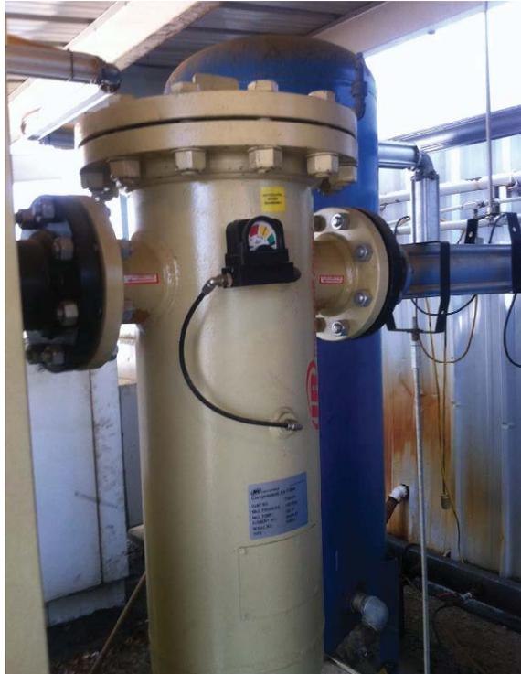
Photo 2: Particulate filter at dryer discharge.
