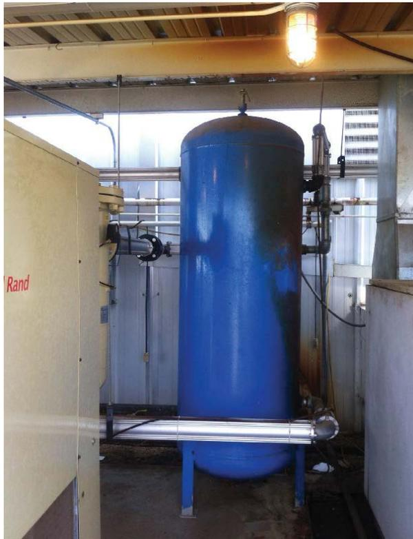
Photo 3: Compressed air receiver.
