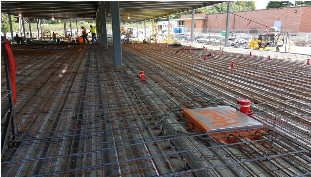
*Slab on metal deck. Manhole opening has candy cane 180 hooks and diagonals.*
