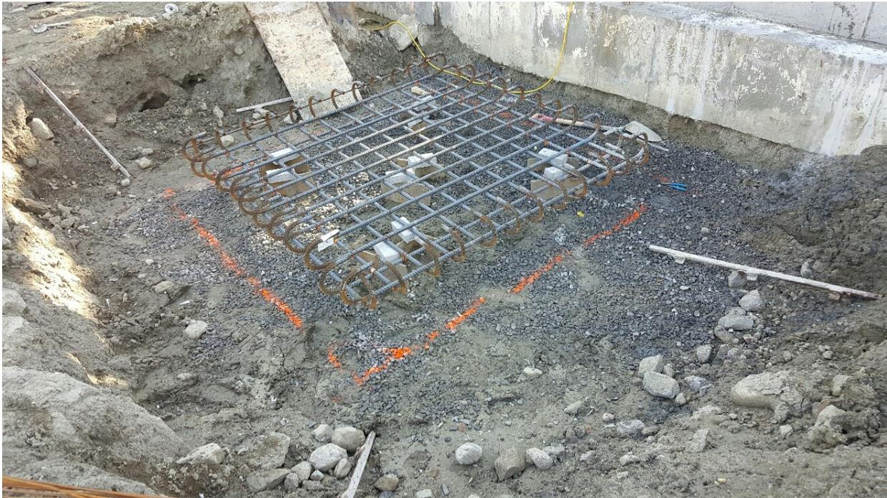
Hooks are governed by the ACI 318-11 Section 7.1 Standard specifying 90 degree hooks have a length of 12 bar diameters (a # 6 hook will have a 9" hook length). 180 degree hooks can vary from 6 to 12 diameters as designed. In the field the iron workers refer to 180 degree hooks as "candy canes".
