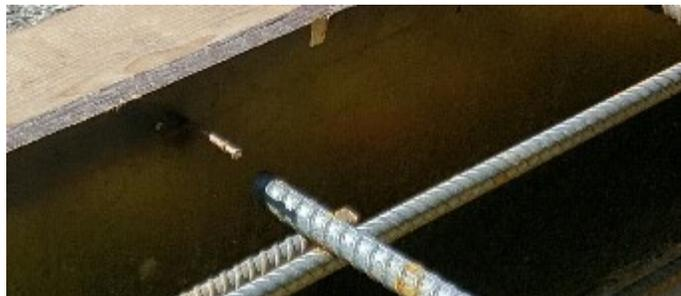
Whether wire fabric or mesh is installed above or below the dowels and any interior rebar, (which will be extra reinforcing parallel to the span direction) is not important. It is the iron workers choice in a thin slab. But attempts should always be made to follow the design drawings unless assembly so impedes. Be sure wire mesh is on chairs and does not simply lie on the metal deck. Chairs should support mesh where it is not near rebar.
