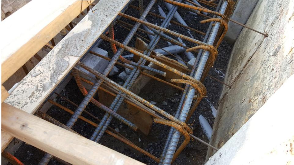
*Grade Beam Rebar with 135 degree bent Stirrups over a Pile*
