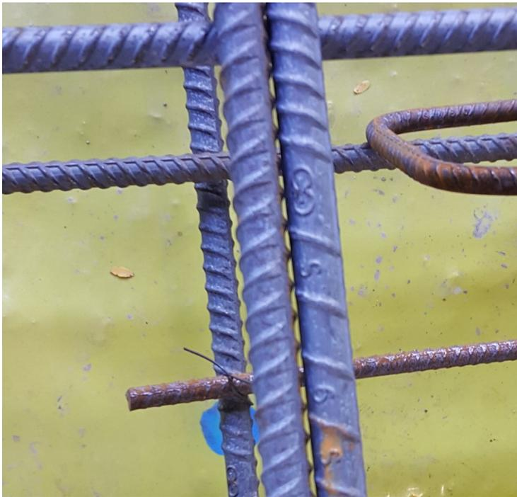
The experienced inspector can instantly recognize the difference between #5 and # 6 rebar without reading its stamped imprint marking.
