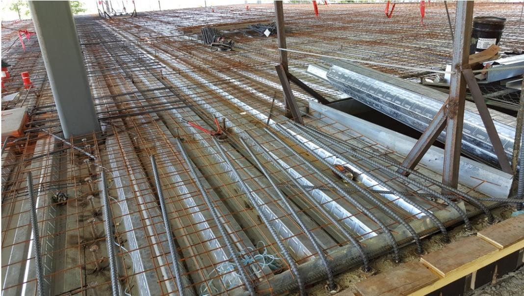
*Perimeter dowels bent down and to be strapped  $\frac{3}{4}$ " below floor elevation*
