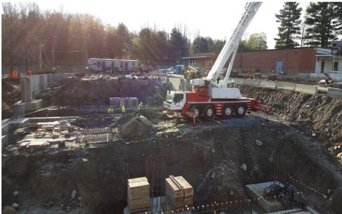
With the rebar cage suspended above by crane, special safety precautions must be taken by the iron workers when slipping the bricks back on the piles to support the rebar weight and give it clearance. Cranes moving heavy objects can be quite silent. If the inspector cannot see the crane operator or the worker directing the operator, they might not see the Inspector, so be aware of crane work.
