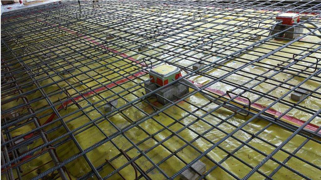
*Slab with grade beams in lower left and upper right. #6 at 12" in direction of span. Utility boxes are mounted on big 4000 psi blocks. Rebar on 4000 psi bricks.*
