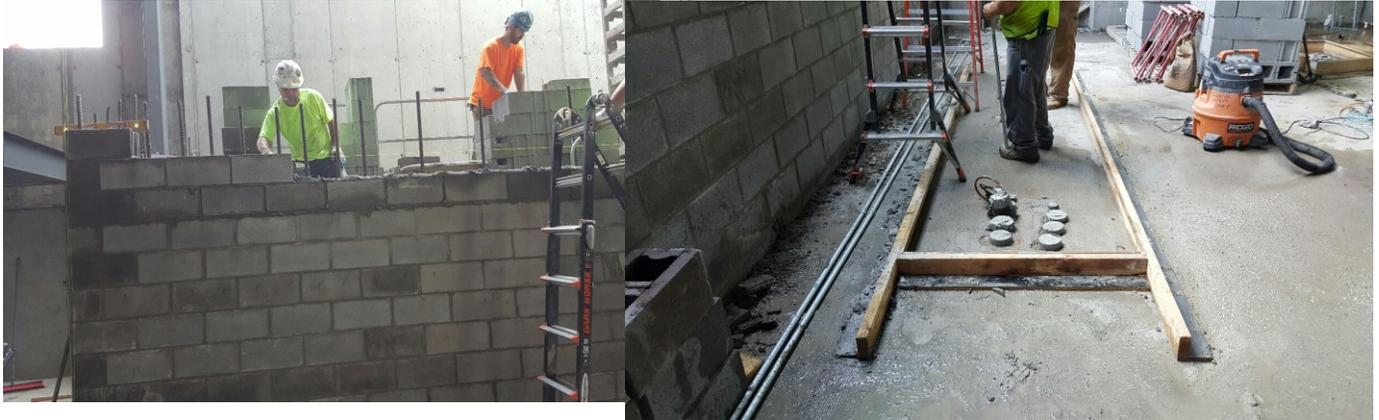
*Masonry dowels were inspected from below before the concrete beneath was poured.*
