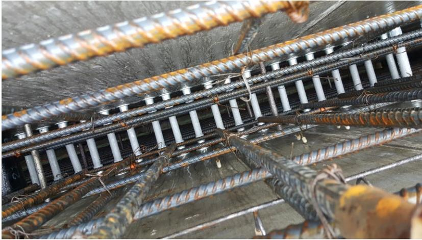
For larger walls, both faces must be inspected for completeness before the second form is placed. Trying to look down a deep form with flashlight is unacceptable, because lower horizontal bars will be out of sight.
