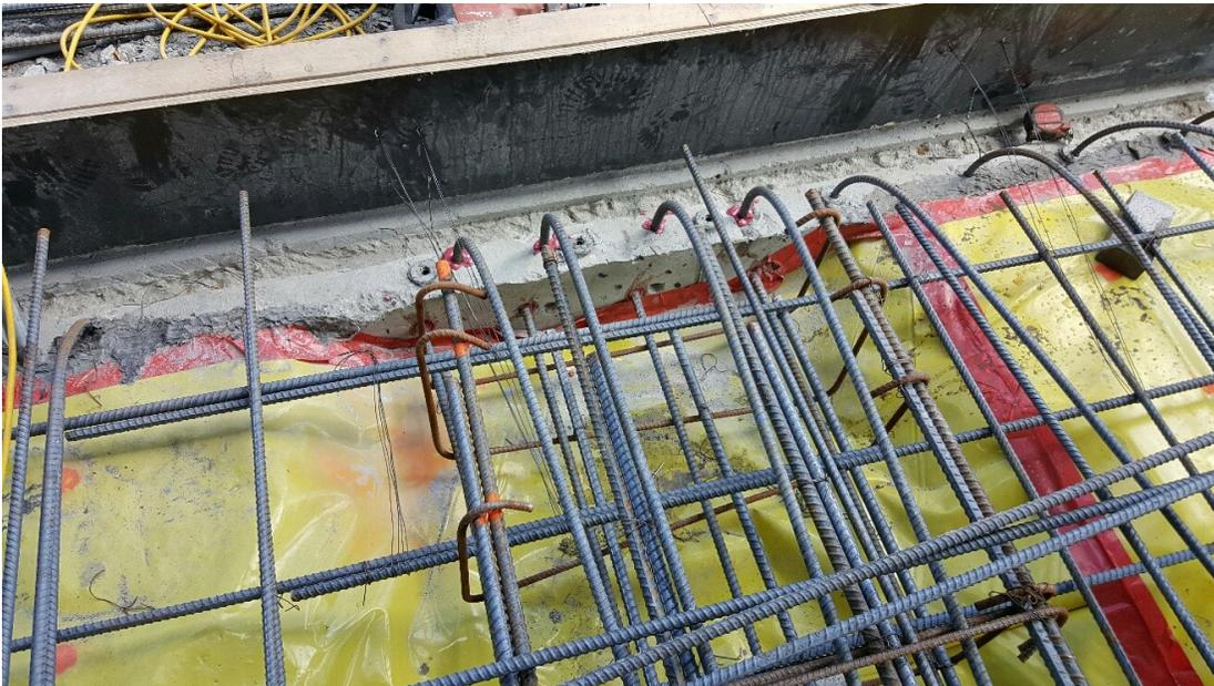
*Dowels as form savers & as drilled and epoxied at slab on grade and grade beam.
