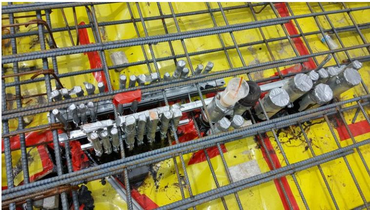
Conduit shown for power and data is not usually in the purview of the rebar inspector. Use common sense when allowing reasonable flexibility in rebar spacing and location.
