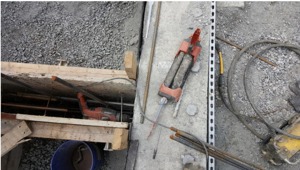
*Drill in place and epoxy gun tool similar to caulking gun ready for rebar insertion.*
