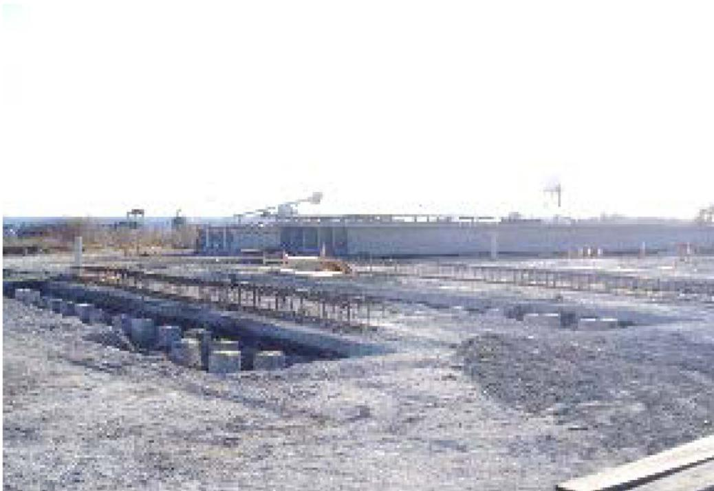
The foundation for the casting cell will need to support at least three segments (which can weigh around 100 tons each), the steel formwork for the segments, the handling equipment used to move the completed segments, and other live and dead loads. The
