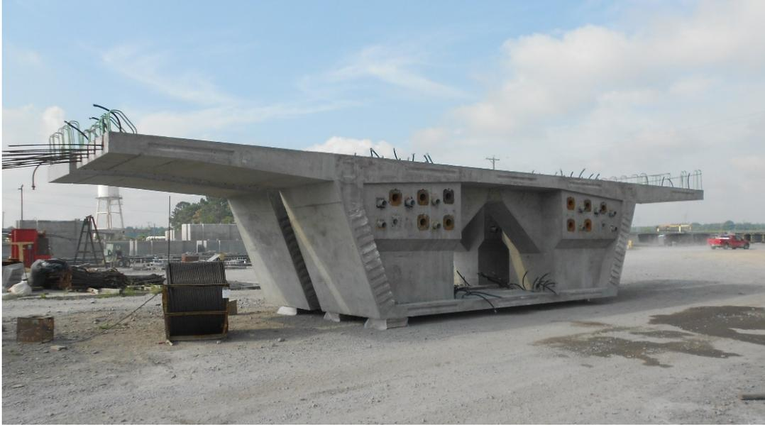
The above completed pier segment show anchor heads and metal ductwork in the cross-section face of the segment and shows transverse strands extending out the wings for stressing
