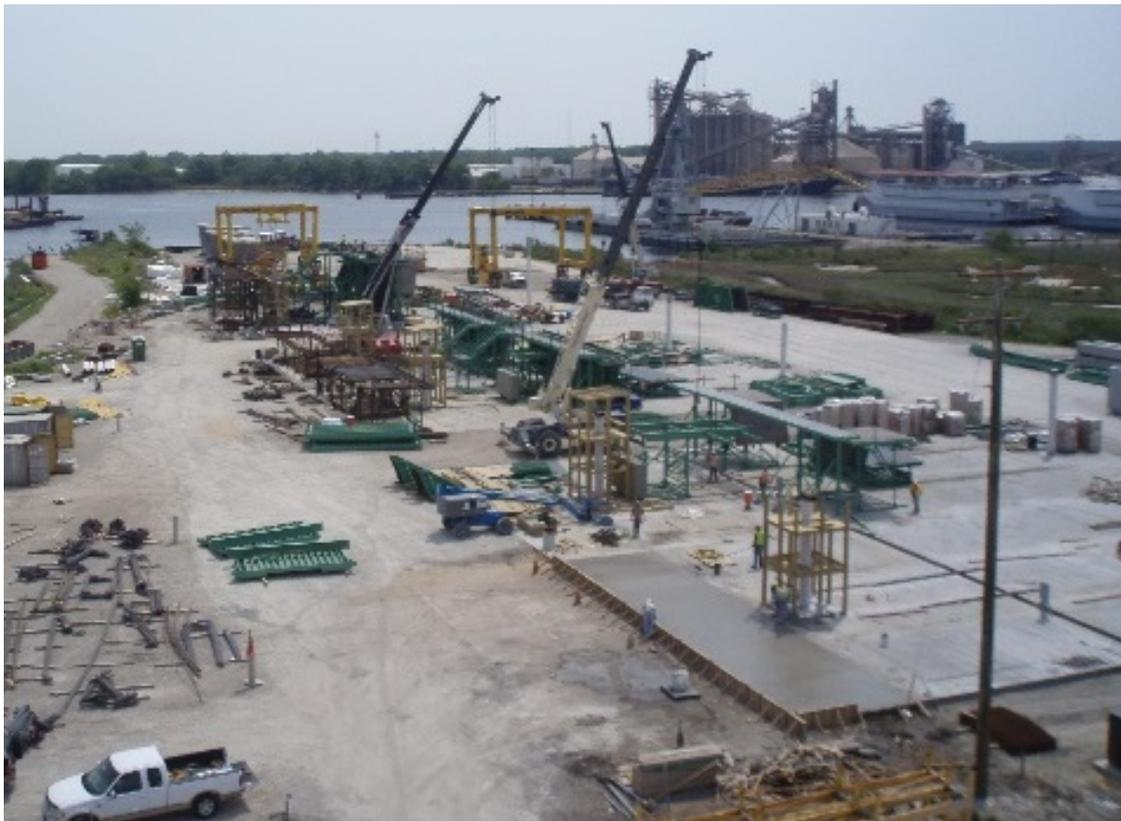
After construction of the footings, the above picture shows casting cells in various stages of completion. The farthest cell is already in production with the straddle lifts moving the already cast segments, the next two cells are near completion with rebar jigs and formwork in place, the fourth cell has formwork and shoring being erected by crane, and the fifth cell's concrete working slab has just been placed and finished.
