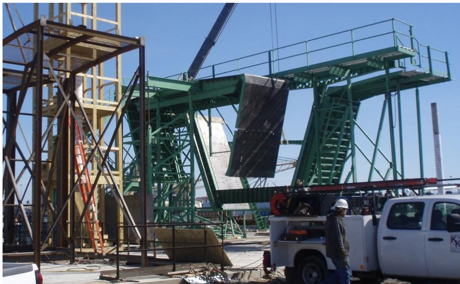
The interior form, or core form, provides the interior opening within the segment. The form supports the segment's interior top slab and controls the concrete thickness in the webs. For ease of stripping the forms after segment casting, the form sides should collapse and the whole system needs to travel in and out of the cell. In order to travel in
