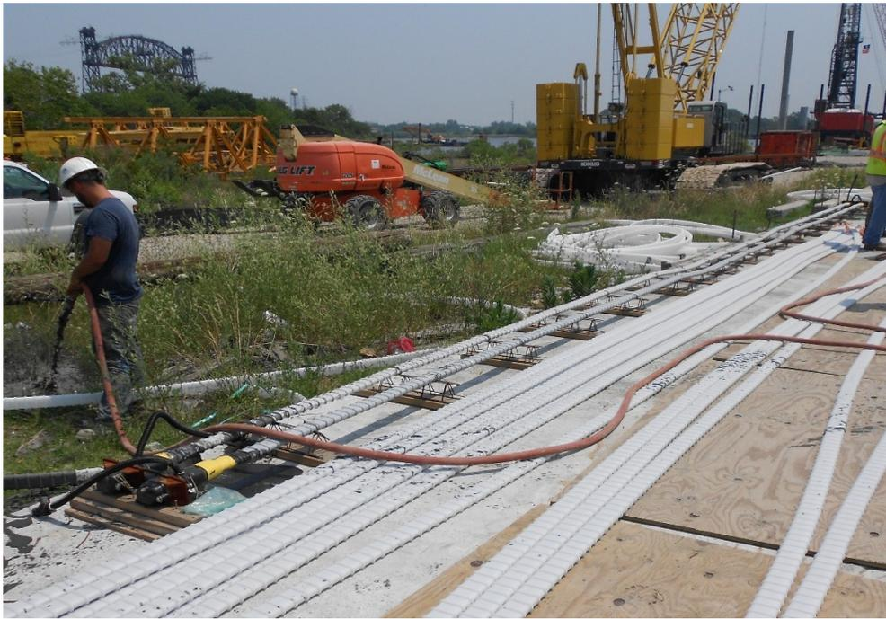
Preassembling transverse post-tensioning duct & anchors for installation in forms
