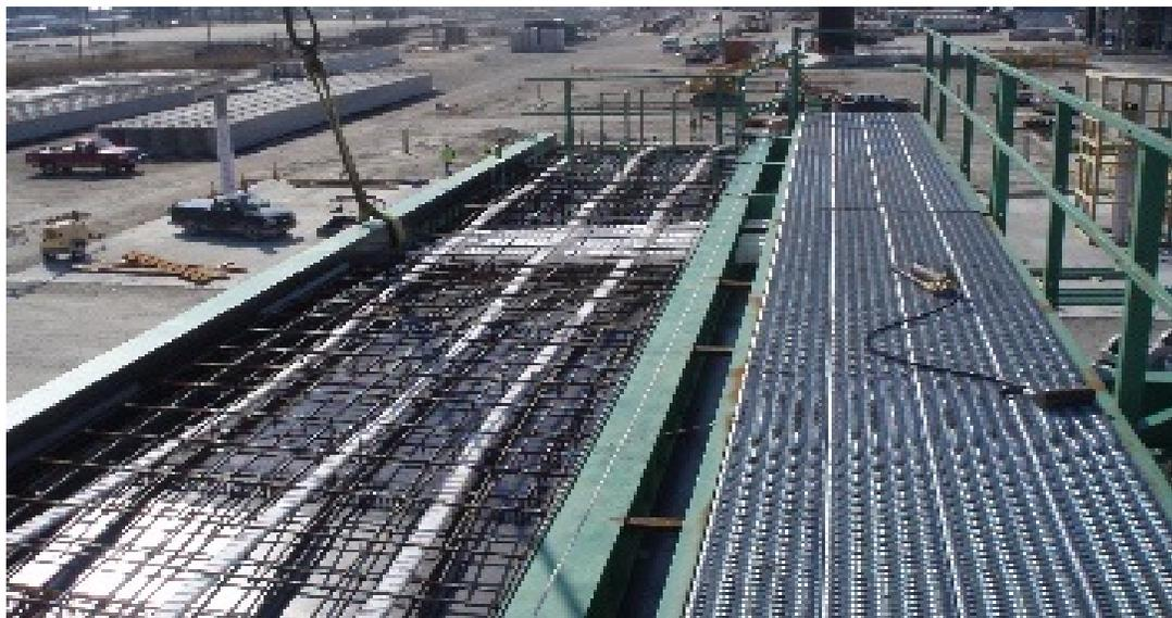
Transverse ductwork installed for a segment prior to placement of concrete in the cell
