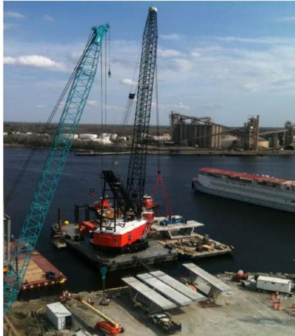
Gantries lifting segments using under wing straps with softeners at the concrete edges
