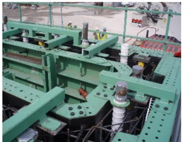
Vertical ductwork for a precast column segment prior to placing concrete in the cell
