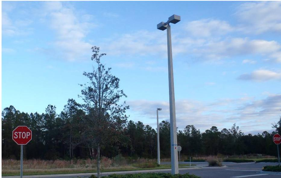
*Site lighting with restrictive down lighting to minimize "light spillage"*
