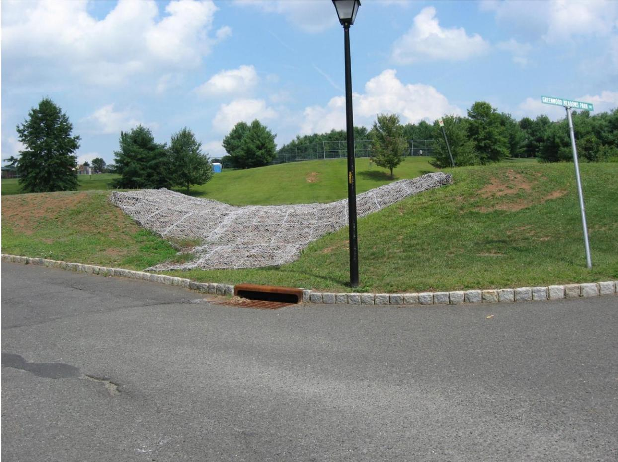
The photograph below shows the same detention basin. The principal spillway (controlled outlet) is shown to the right and the armored emergency spillway is shown to the left of the photo. Note that the controlled outlet has an open top (with a trash rack to collect debris and for
