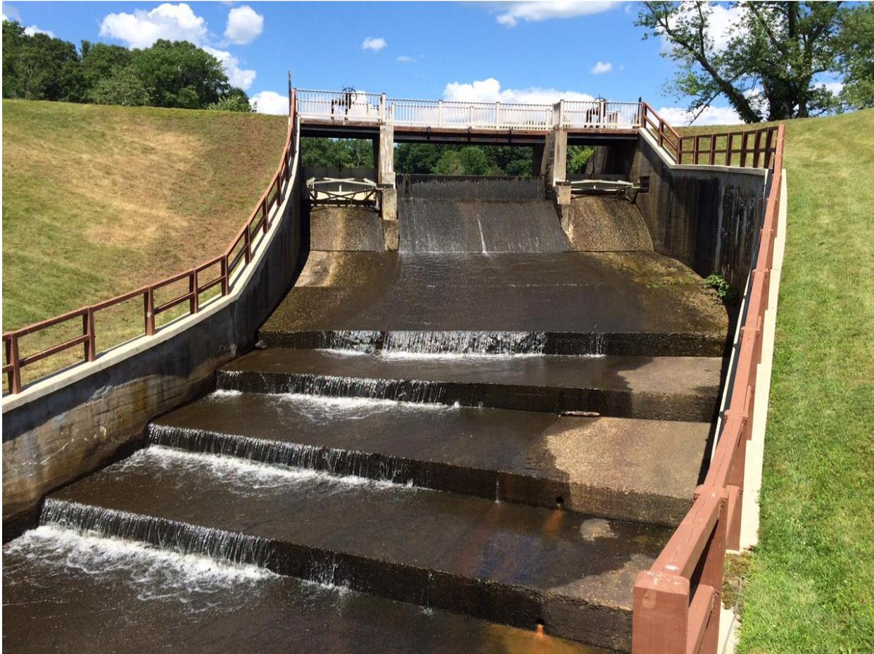
This dam spillway was constructed many years ago and serves a pond that is used for recreation purposes by a residential homeowners association. It can be seen that this spillway is properly functioning, well-maintained, and non erosive. These features must be built into the design of and dam spillway, no matter what the size of function of the pond.
