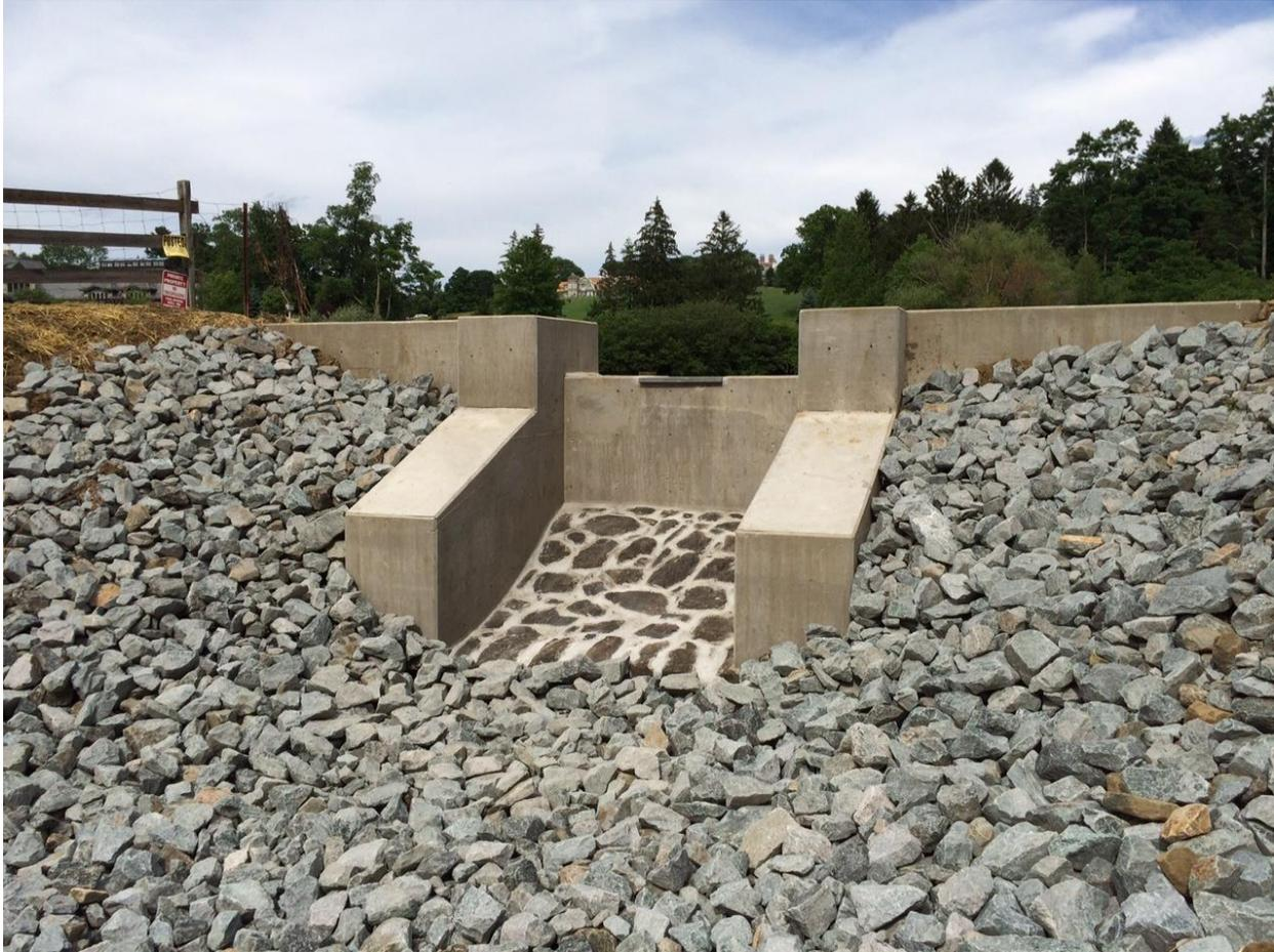
To calculate the flow through the spillway structure it is important to determine the type of structure and correctly model the outlet. Many spillways function as some type of weir. The most common types of weirs are as follows:
