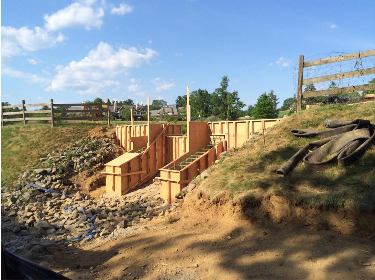
In order to set the forms shown in the photograph above, it was first necessary to carry out dewatering operations, bypassing this area with the outflow from the pond.
