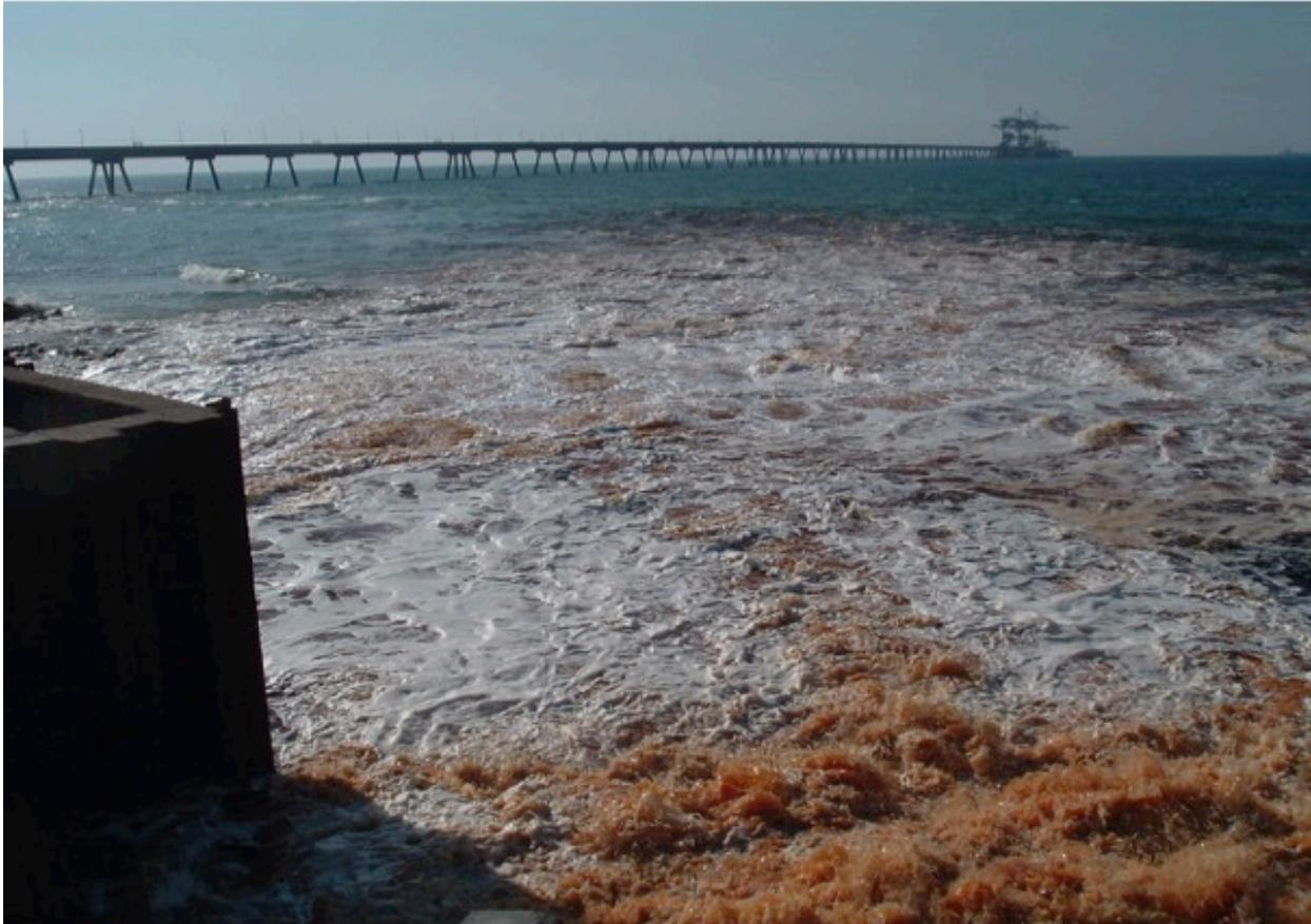
**Figure 10 – Desalination Plant Discharge with Elevated Iron Content**
