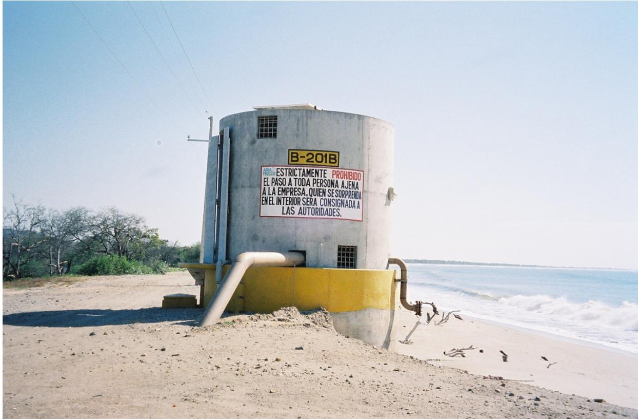
**Figure 8 – Radial Intake Well of Large Seawater Desalination Plant**
