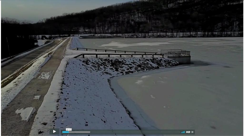
*This Cyclopean masonry dam (named for the only giant who could lift the stone blocks) was core drilled under the author's inspection years ago. Drones will enhance dam inspection in the future.*
