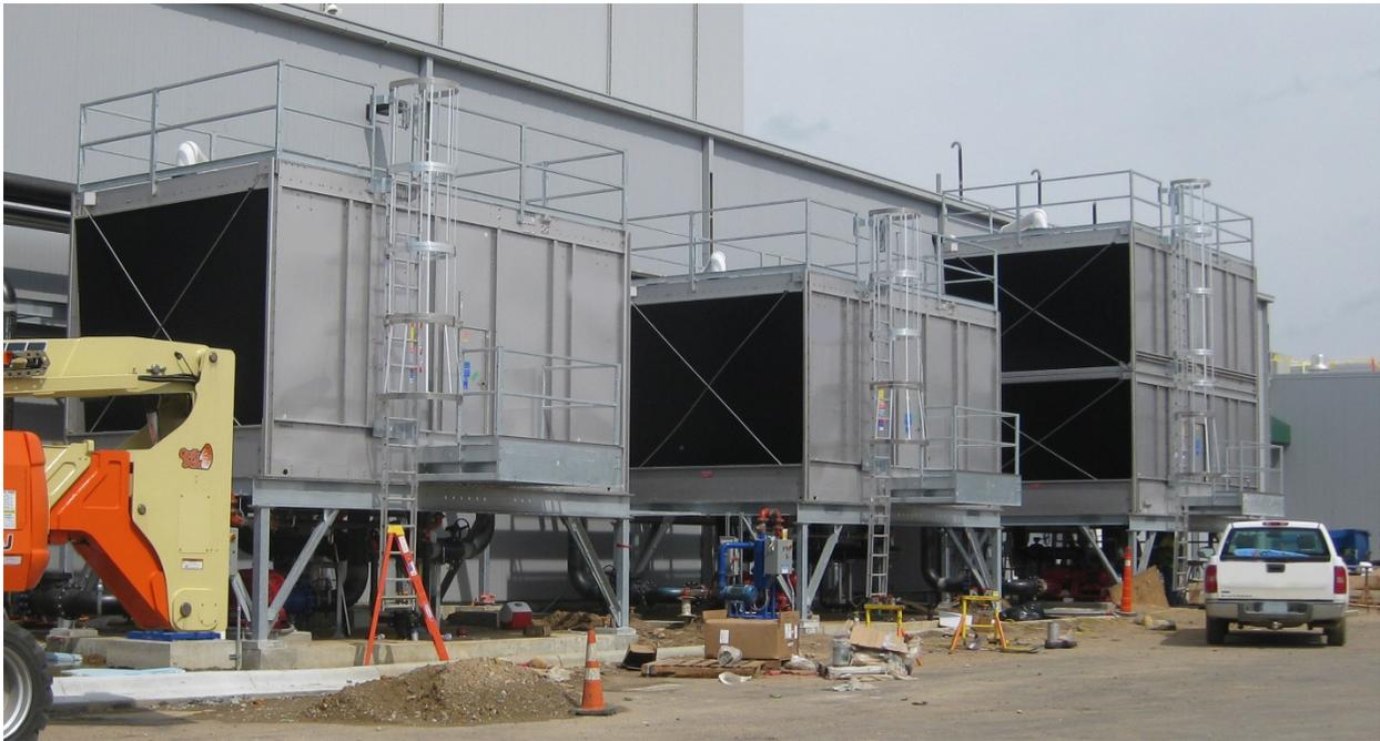
Figure 16: Elevated Cooling Towers with Condenser Water Pump located Beneath
