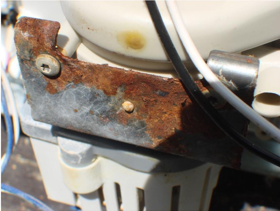
Photo #37 – This is the same instance in the previous photo seen from below. The heavy corrosion indicates a longer-term leak.
