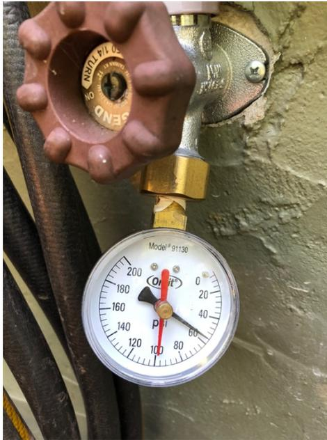
Photo # 3 -- This is an inexpensive pressure gauge used to check the proper function of a pressure reducing valve. Use one with a maximum reading capability (red needle) to determine maximum pressure over a period of time. The red needle is pushed up by the black needle that actually indicates the pressure. This photo was staged – the house is really on well water.
