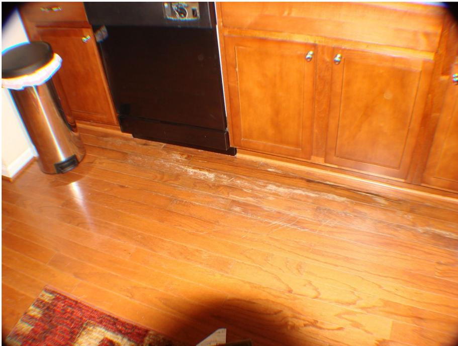
Photo #18 – The water from a leak tends to run under the finished floor towards a low part – usually the center – of a room.
