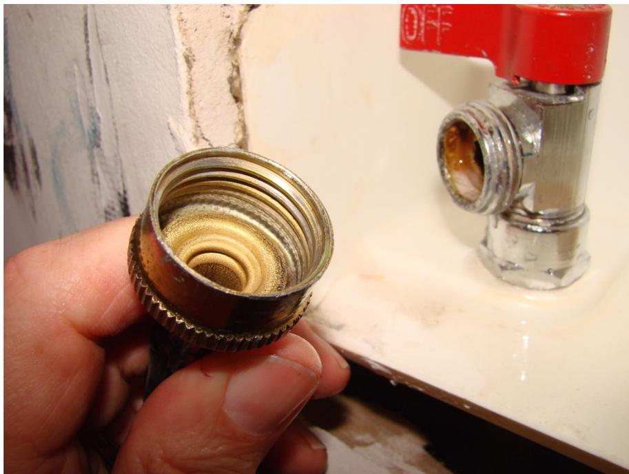
Photo #65 – The issue in this case was a supply hose installed by a rental company that had no washer in it. It leaked through no fault of the washing machine.
