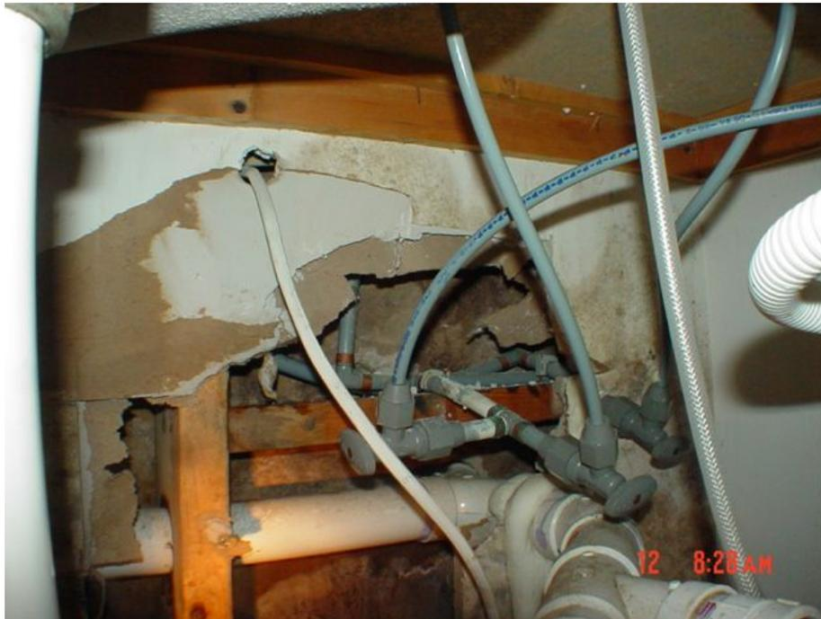
Photo # 11 -- This is polybutylene piping. It is always the gray color and is subject to pinhole leakage, as was this case with this pipe in a confined space.
