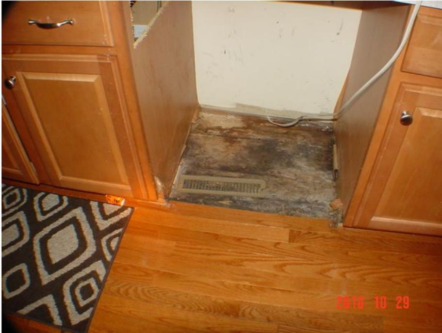
Photo #17 – Typical water staining left after a dishwasher leak. We need to determine the time frame of the leak and this staining assists us in doing that.
