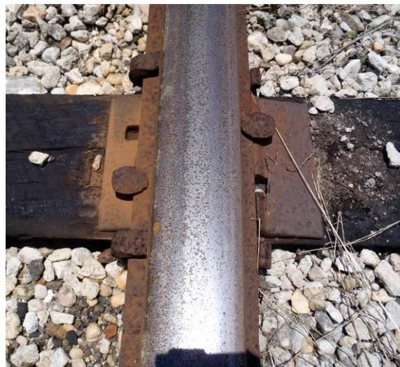
Figure 9 – An installed Tie Plate
