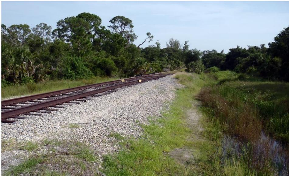
Figure 12 – Railroad drainage ditch to manage stormwater
