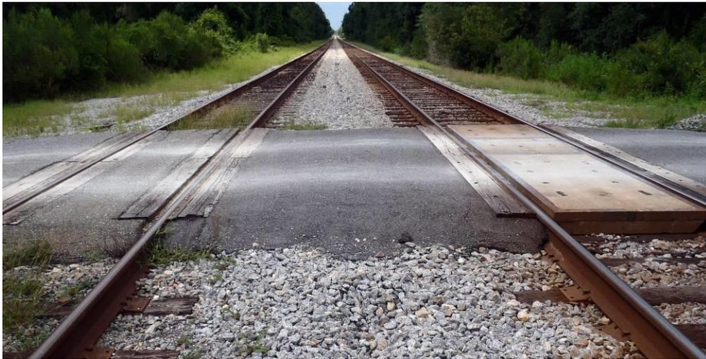
Figure 27 – A rail crossing using asphalt, concrete, & timber materials
