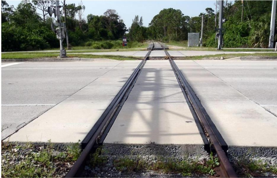
Figure 28 showing a road crossing using concrete.
