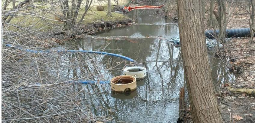
feet in diameter and have a peastone filter around the pump. A 6" diameter pump or one of suitable size will be set in this basin with enough hose to pump from the basin into the bypass swale upstream of sedimentation controls.
