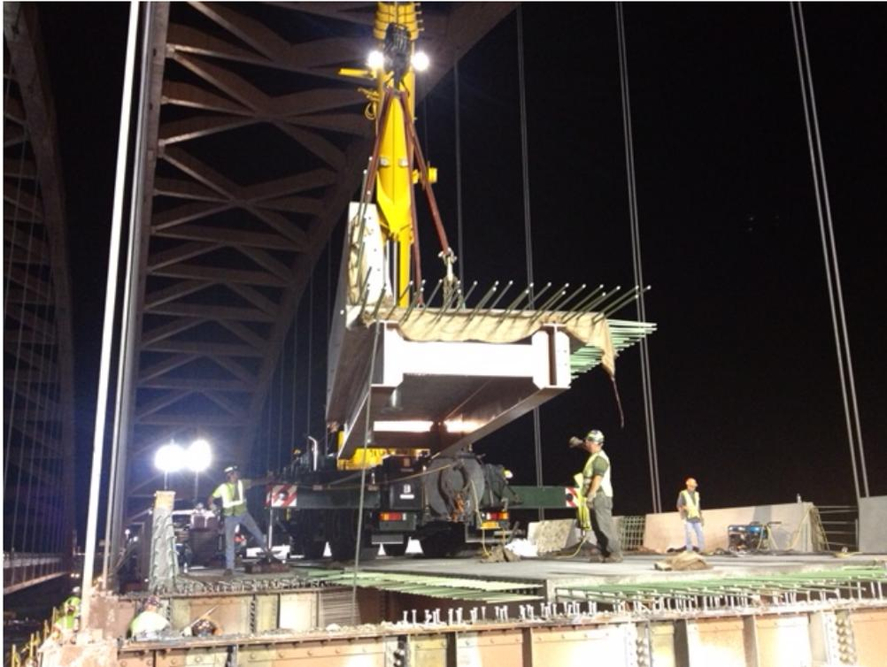
First a crane erection plan - design and working drawing submittal must be put together. The plan will include crane information, rigging and lifting devices, site information including ground bearing pressures and possible obstructions, and traffic control if needed. The sequence of erection will be detailed and any temporary bracing or supports will be shown if the initial erection is not self-supporting.
