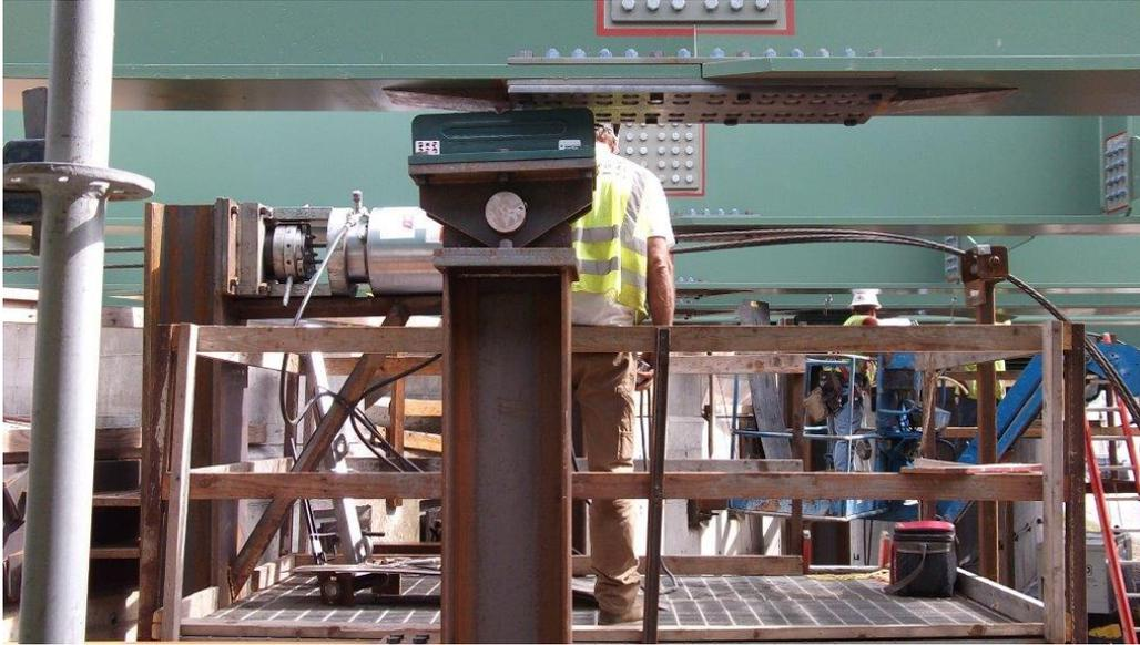
roller bearing support under structural steel with strand jack assembly behind
