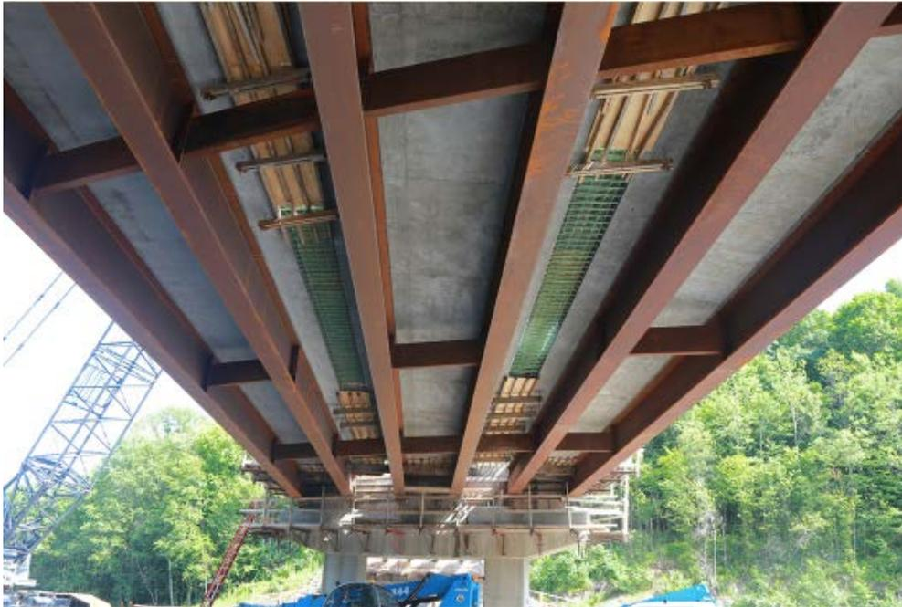
Concrete will be delivered, placed, and finished within a specified time to avoid workability issues with the initial set. High early mixes contain an accelerating admixture that will “flash” set the concrete once activated. Manipulating the concrete after this occurs may damage the concrete surface and jeopardize the durability of the closure pour.
