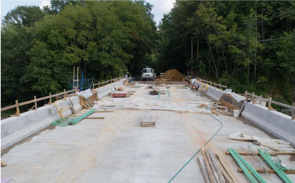
After curing, the finished closure pour concrete surface shall be inspected for cracks. The inspection and any necessary repairs shall be completed prior to the preparation of the deck final surface treatment.
