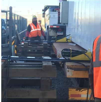
Hydraulic Jacks w/Teflon Sliding – Pushing Trays
