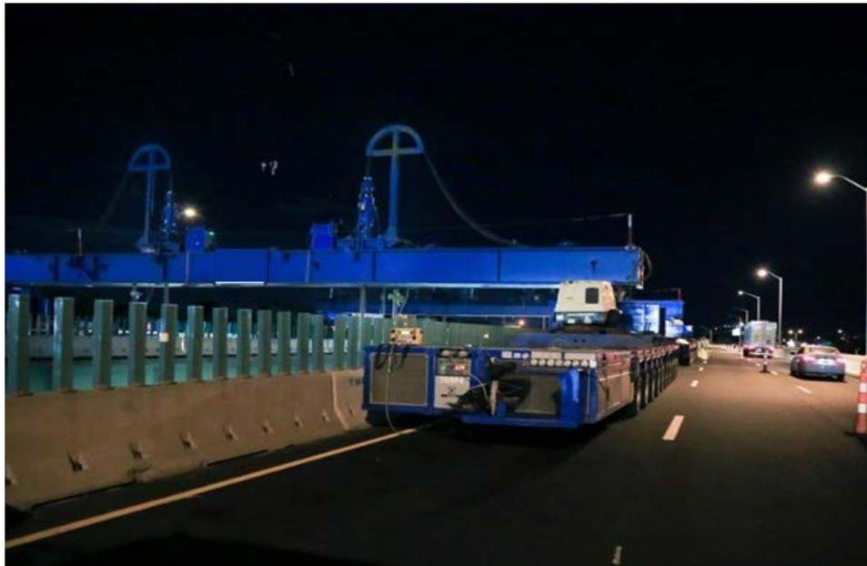
SPMT move median PBU span held with carrier beam and strand jacks
