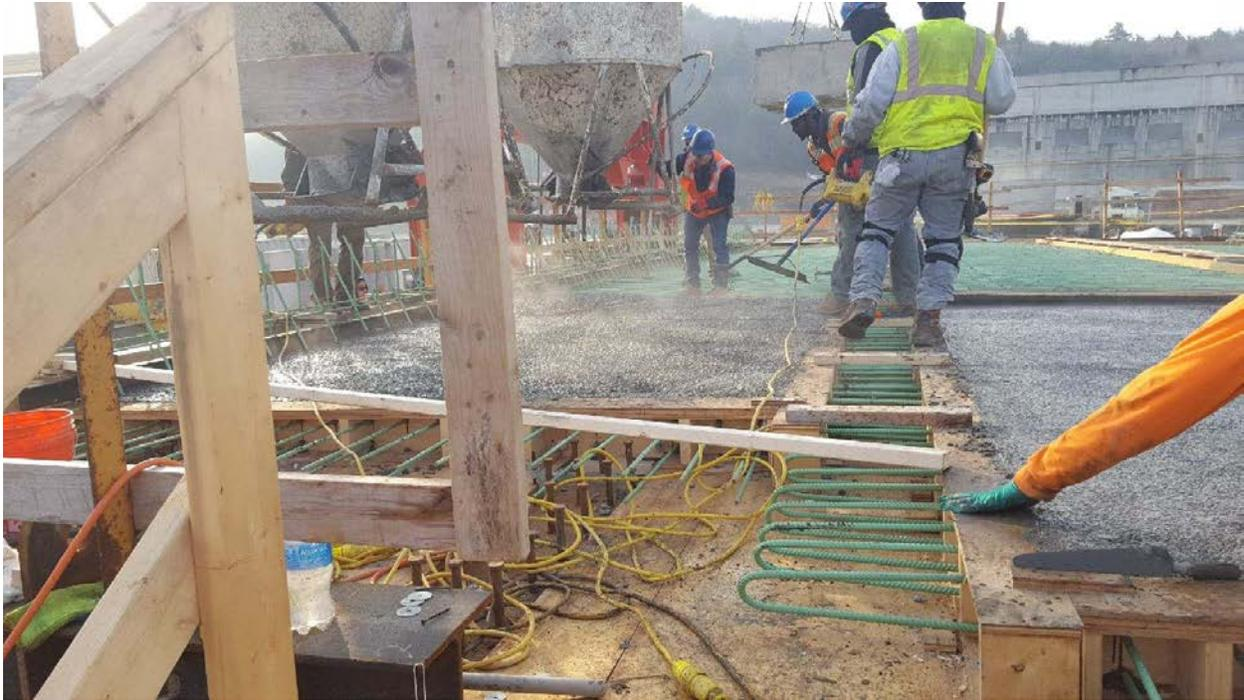
Before and during the concrete placement, quality control tests must be performed both at the plant for production and at the placement. Air content, temperature, and slump testing, plus the casting of concrete cylinders for laboratory compressive strength testing are the minimum tests needed to ensure a quality cast.
