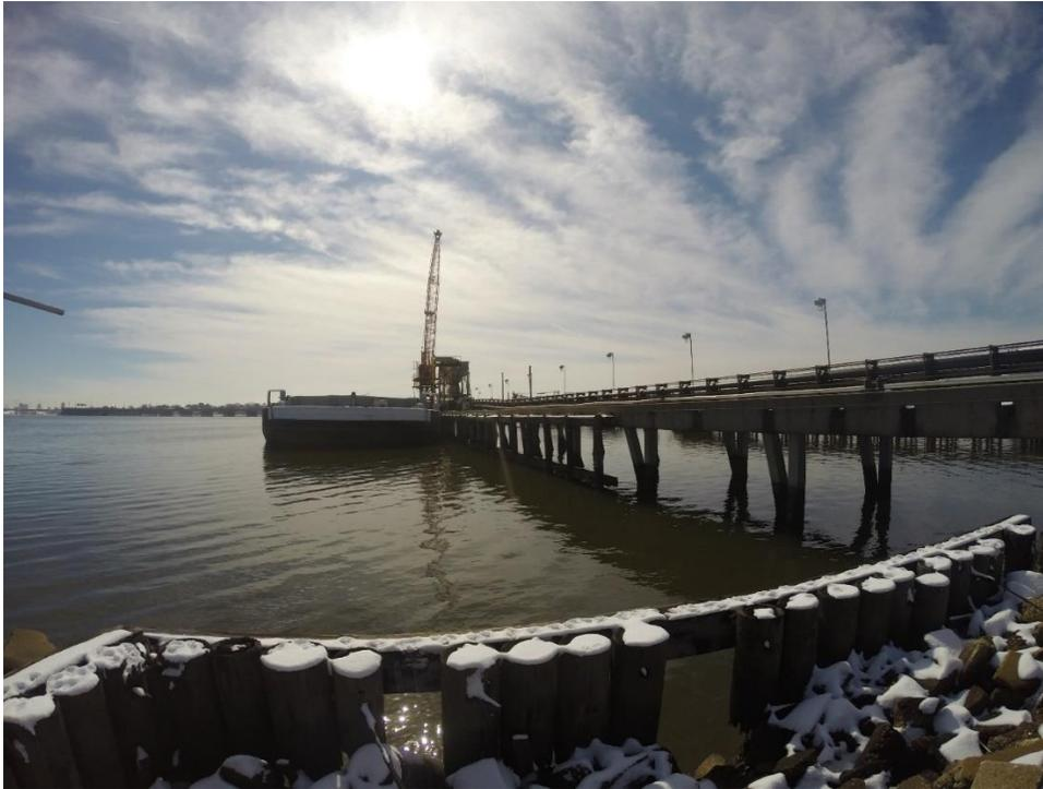
This image shows a pile supported pier extending out into deeper water and a waterside crane that can be used for loading and unloading vessels.
