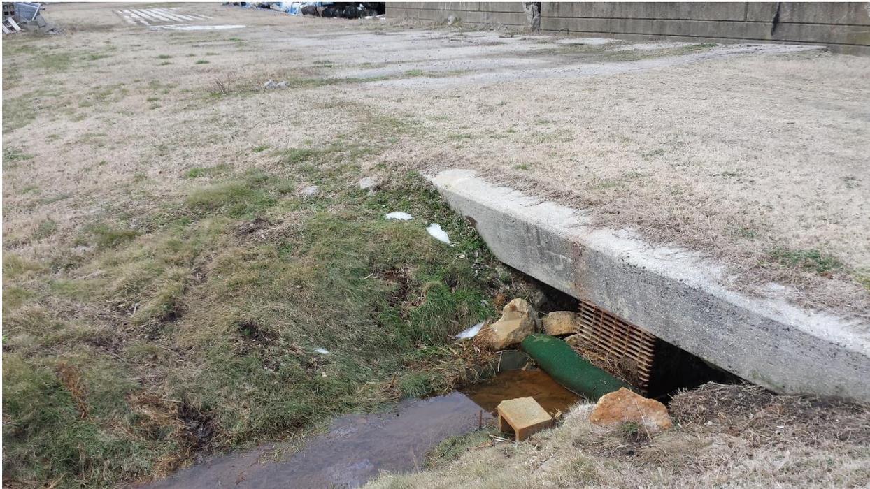
This image shows a stream/swale passing underneath a concrete structure, which indicates traffic passes over the bridge. The stream/swale has a wattle/sock and a steel grate over it, indicating there may have been debris blockages or environmental releases in the past.
