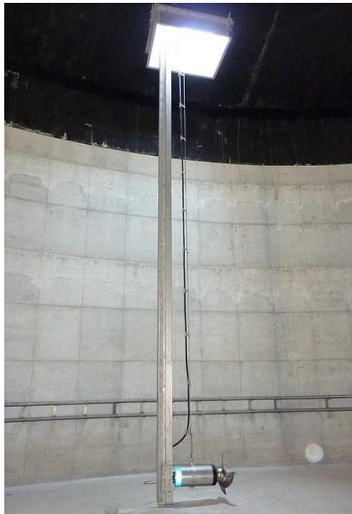
Figure 10: A rail-mounted submersible mixer which is removable from the hatch above.
