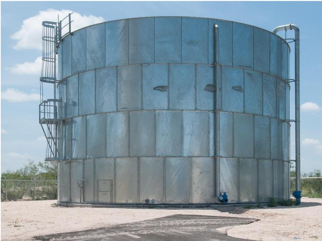
Figure 1: A stainless steel ground storage tank
