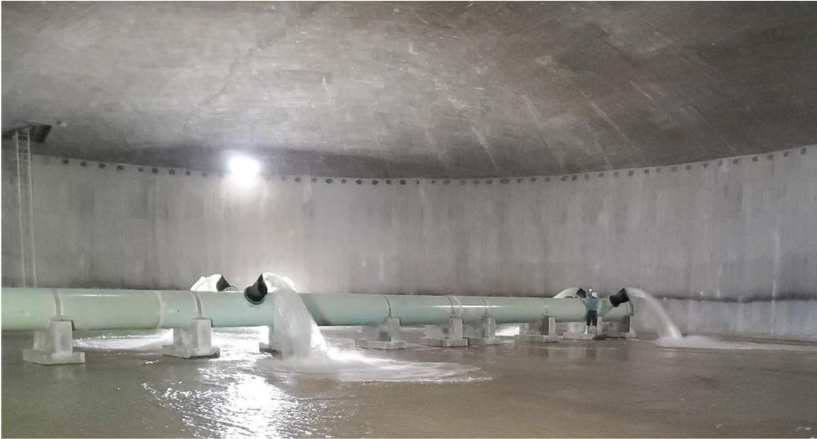
Figure 9: A passive mixing system with several nozzles designed to mix the entire tank.
