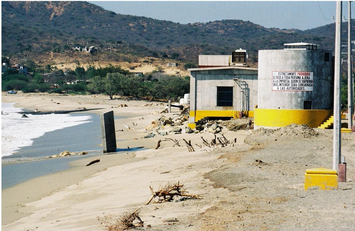
**Figure 2:** Seawater Intake Well Exposed to Beach Erosion
