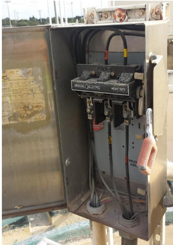
Figure 25: A 30-year-old disconnect switch on a clarifier.
