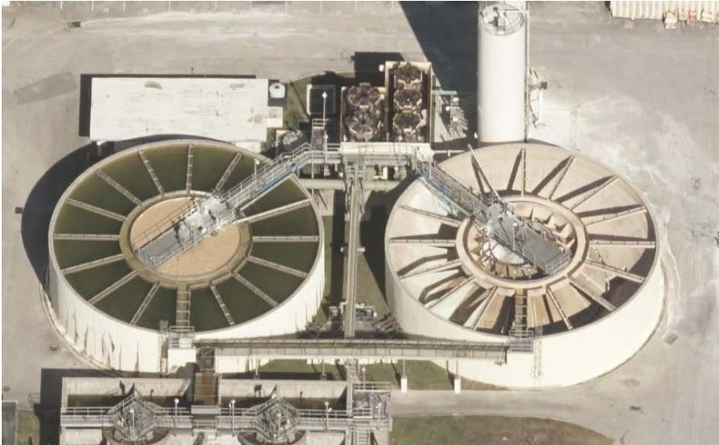
Figure 10: Example of two solids contact clarifiers for lime softening of water. Raw water is pumped into aerators (in the center) and then flows by gravity to the two clarifiers. Effluent flows by gravity to sand filters. The lime silos can be seen behind the empty clarifier.
