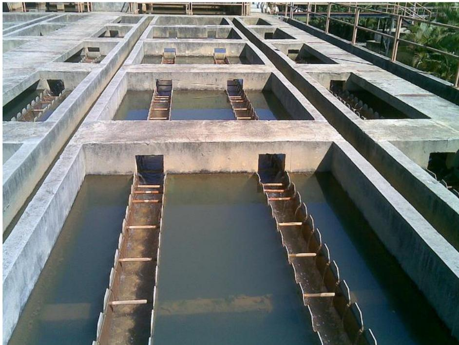
Figure 7: Rectangular clarifiers with effluent troughs.
