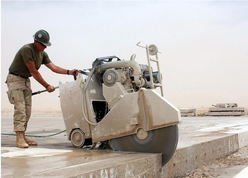
Fig. 21 - Sawcutting a concrete slab (Source: [http://www.navy.mil/view\\_image.asp?id=24454](http://www.navy.mil/view_image.asp?id=24454); Author: Mark H. Overstreet)
