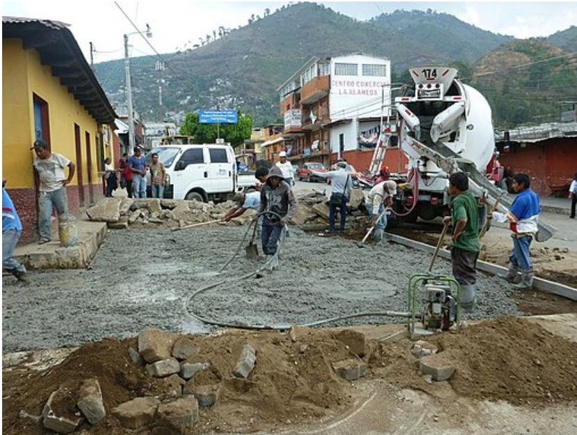
Fig. 12 - Wet concrete being placed – [mardoqueo sagastume / CC BY (<https://creativecommons.org/licenses/by/3.0>)]
