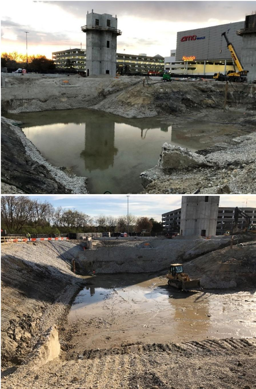
Fig. 6- Site groundwater – before and after de-watering – 2,700 gpm constant flow. High water table forced the owner's design team to use a mat foundation 5 feet thick to counteract the hydraulic pressure beneath the waterproofed basement.
