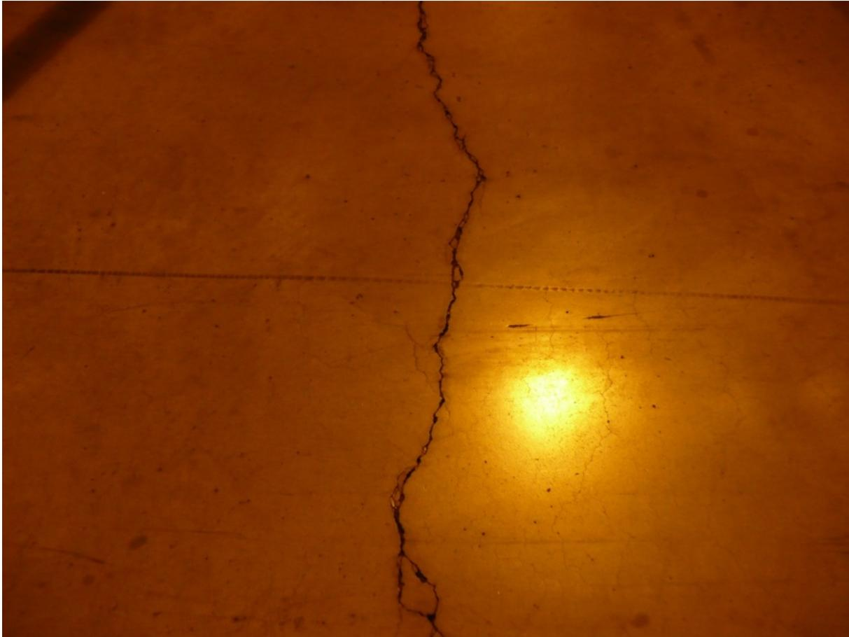
Fig. 31 - Typical random crack in concrete slab
