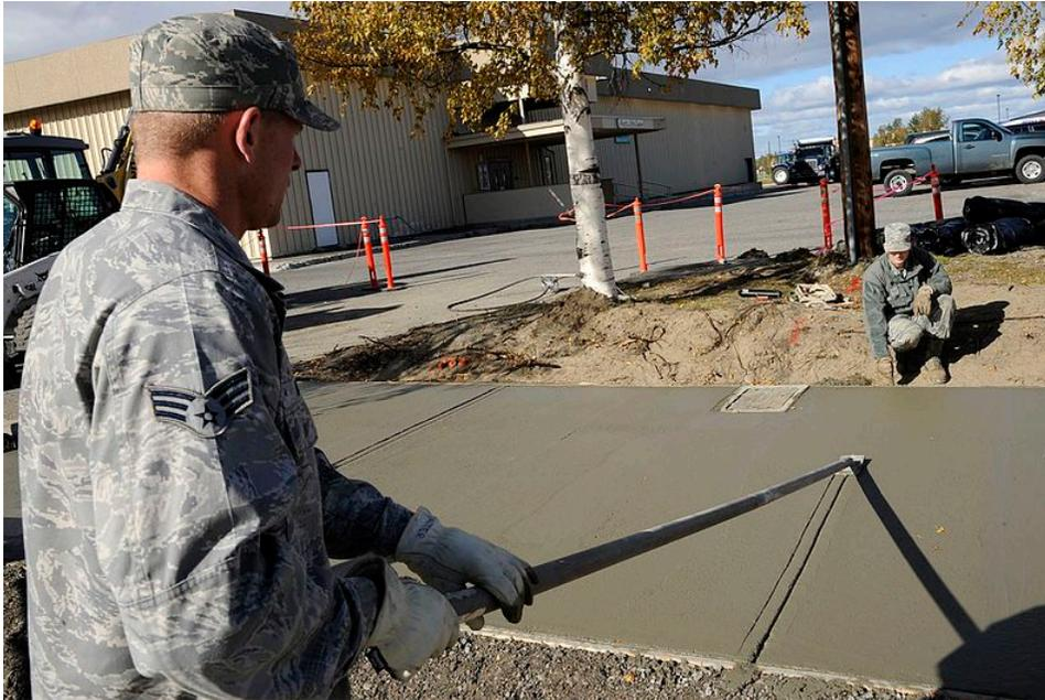
Fig. 23 - Tooling joints in a concrete slab – (Source: <https://www.dvidshub.net/image/664009/dirt-boys-pave-eielson-streets>; Author: Staff Sgt. Jim Araos)
