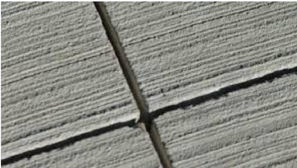
Fig. 22 - Typical final sawcut in concrete slab
