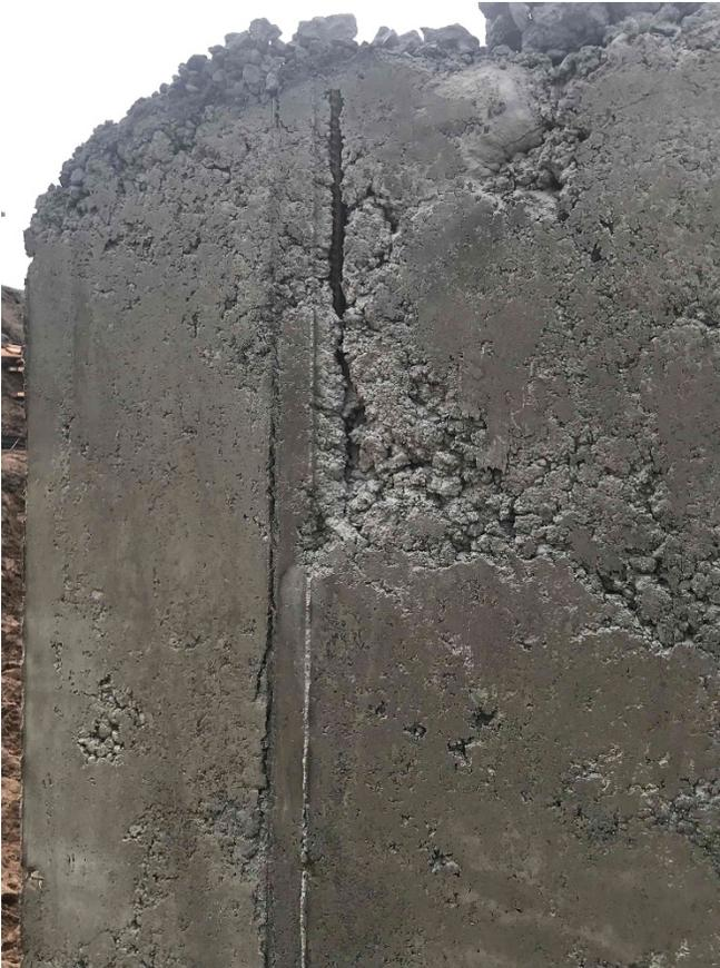
Fig. 13 - Honeycombing –Poorly vibrated concrete
