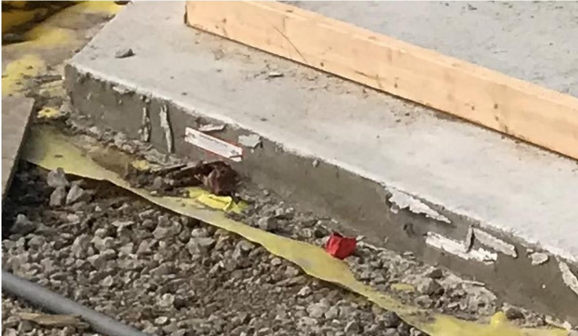
Fig. 30a – Insert at edge of construction joint set into first concrete pour, with second concrete pour to follow
