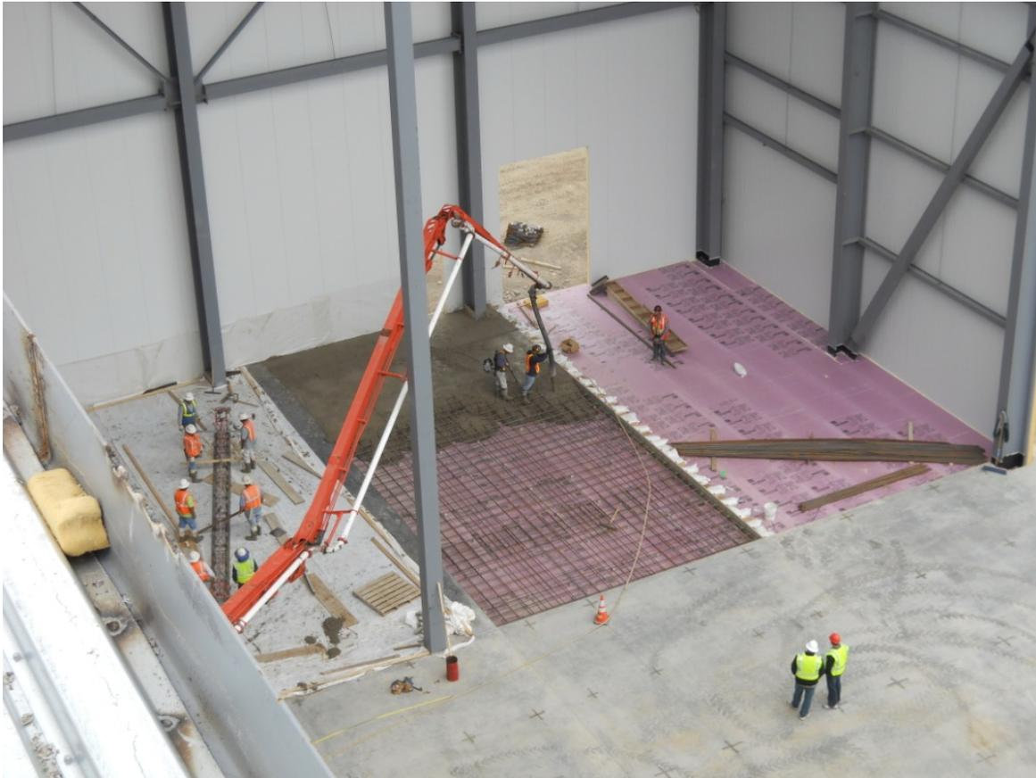
Fig. 2 – Slab-on-grade being poured for a freezer warehouse, with optional reinforcing
