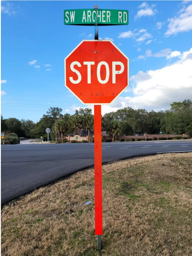
Figure 21. Reflective material on sign support
