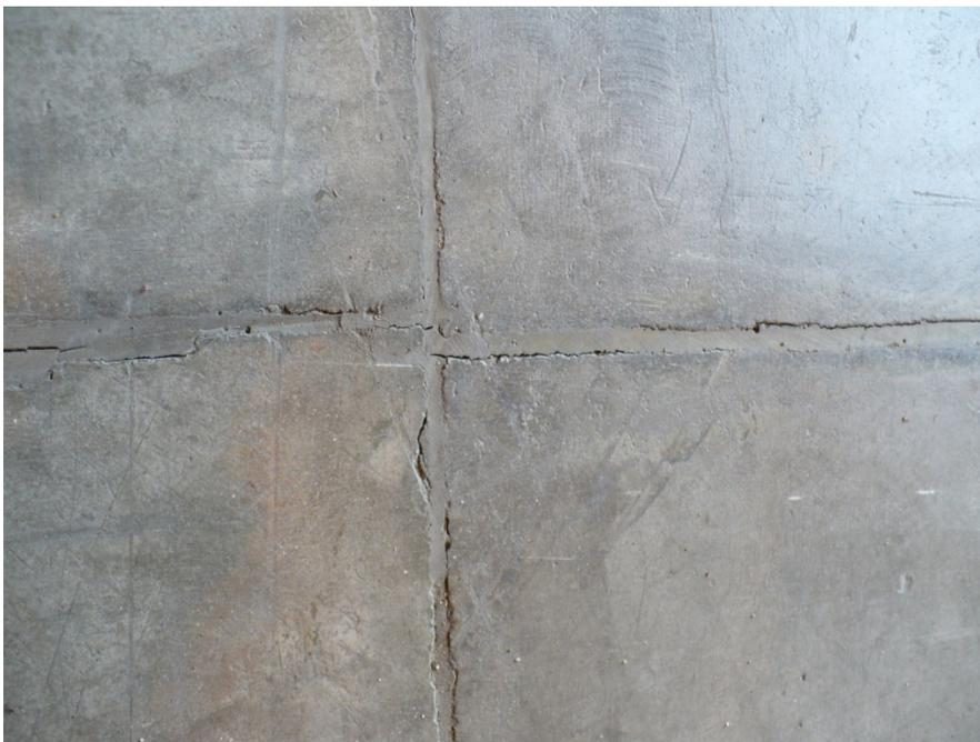
Fig. 50 - Joint filler in slab joints
