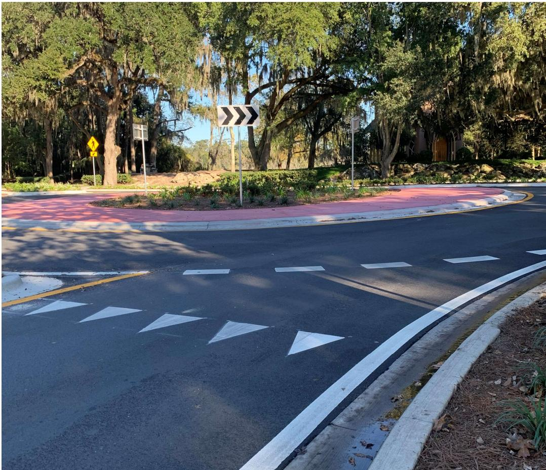
Figure 21. Roundabout approach marking
