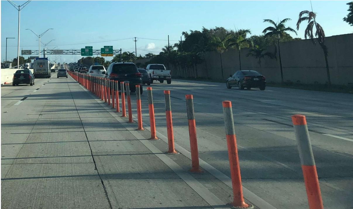
Figure 31. Lane divide channelizing devices
