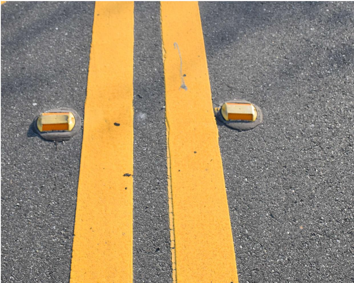
Figure 11. Yellow double line markings with pairs of RPMs
