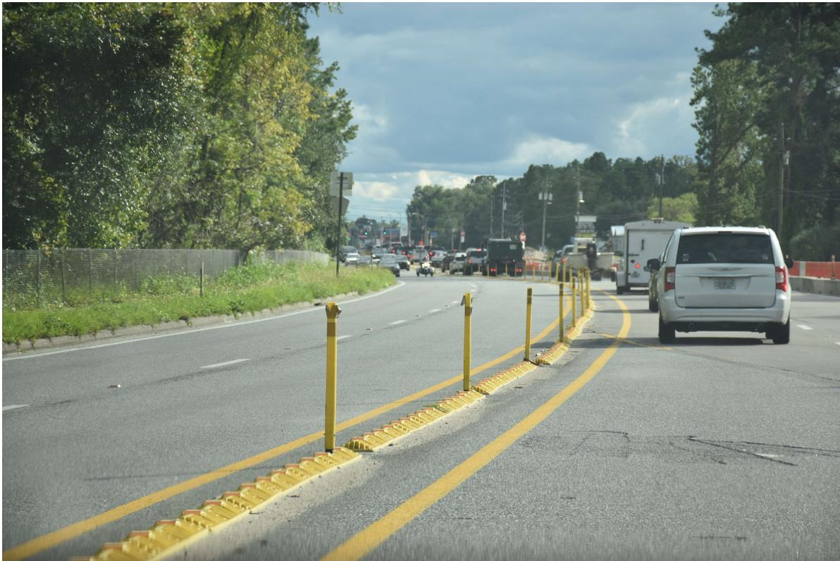
Figure 30. Center line channelizing devices
