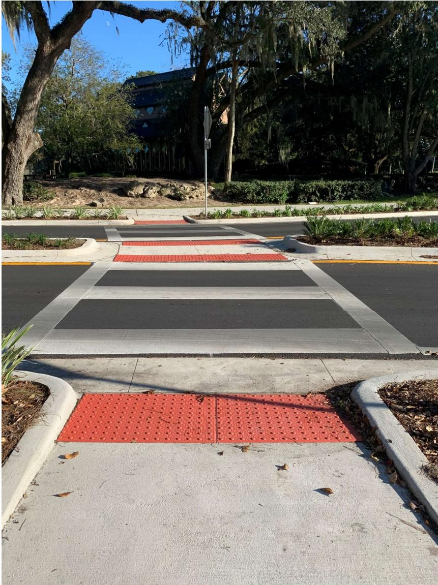
Figure 33. Pedestrian detectable warning surfaces
