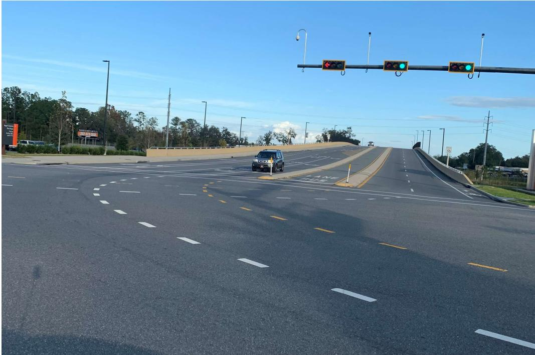
Figure 8. Dotted-edge lines extended through intersection
