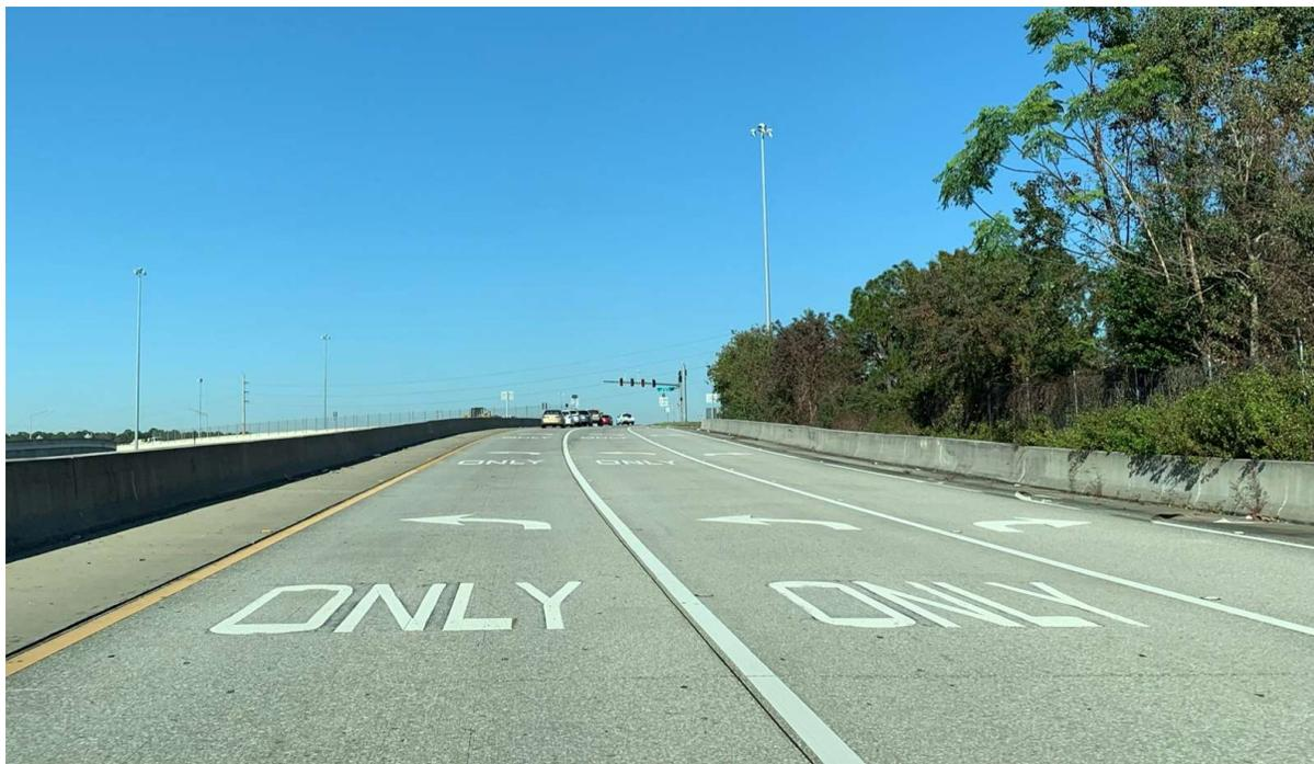
Figure 18. Word and arrow pavement marking
