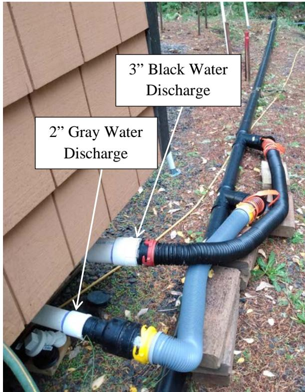
**3" diameter RV hoses with "bayonet" style connections connect this THOW to ABS piping that discharges to a septic tank. The gray and black water from the THOW is mixed since the septic system can treat both.**
