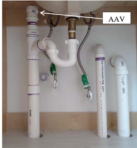
**Drain pipe (left) and two vent pipes (middle, right) located inside the bathroom vanity of a THOW.**
