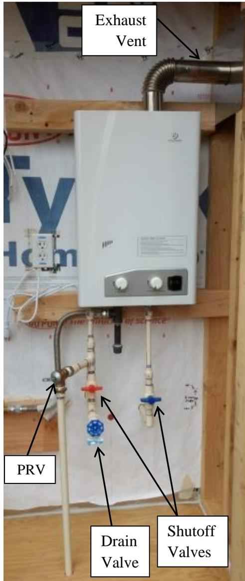
**A tankless, or on-demand, propane water heater installed in a THOW. This water heater model plugs into a 120 volt electrical receptacle to power the flame igniter. Models with battery powered flame igniters are also readily available.**
