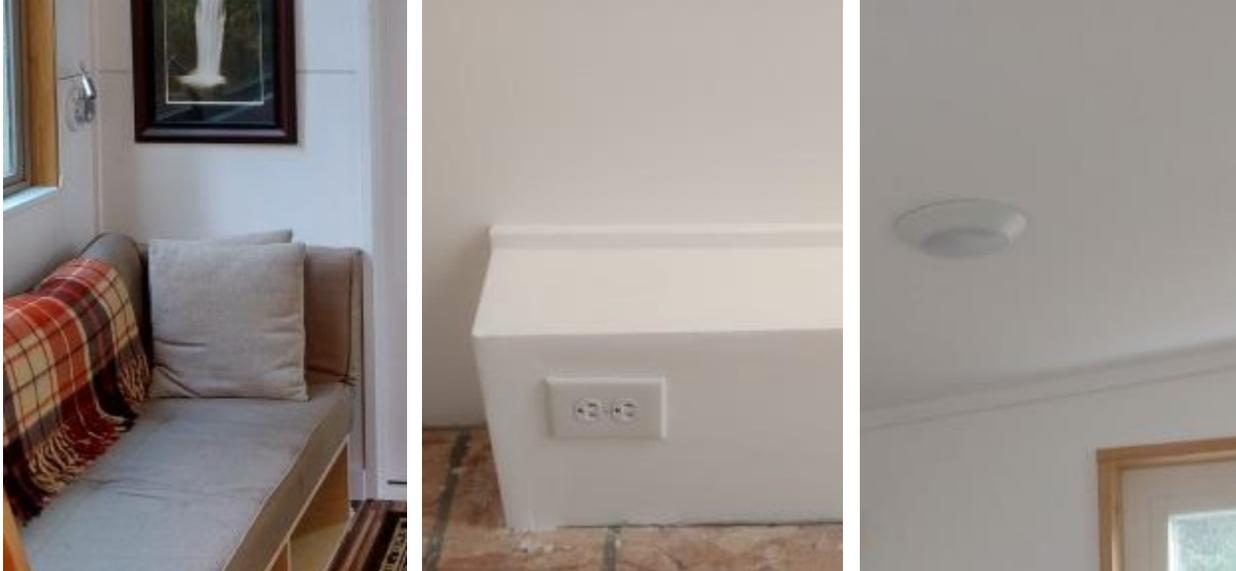
**Left:** A flexible gooseneck, wall-mounted, 3 watt LED reading light in a THOW. The light has an on/off switch located on the lamp base and was hardwired to the electrical circuit to avoid the clutter of a cord.
