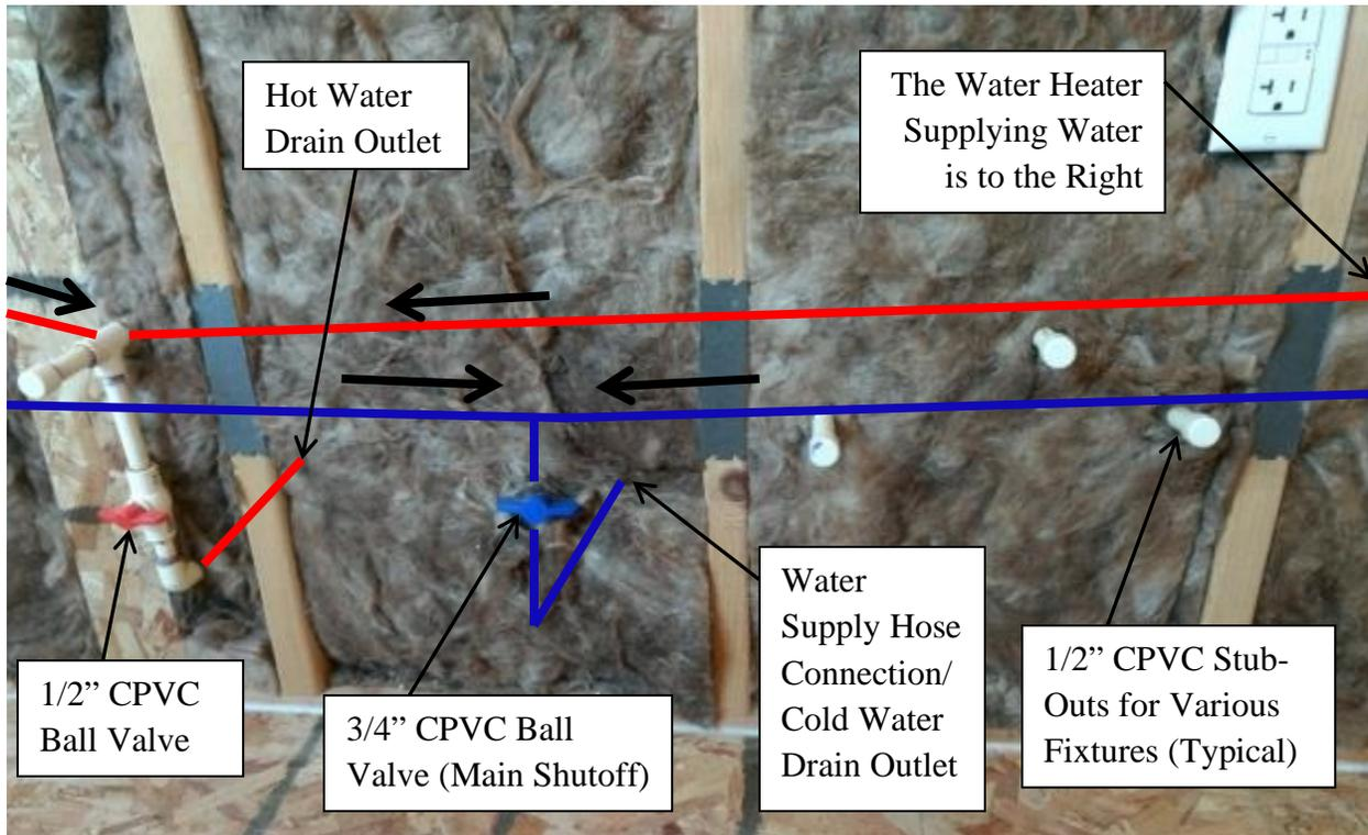
**The hot water and cold water pipes each slope to a low point in this seasonally used THOW. The 3/4" cold water ball valve is normally open while the 1/2" hot water ball valve is normally closed. Each autumn the water supply is turned off, the hose is disconnected, and the hot water valve is opened. Both hot and cold water drain out by gravity onto the ground. Both valves are then closed for the winter.**
