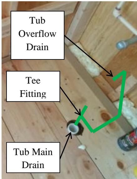
**Bathtub main drain and future overflow drain (green lines) configured to avoid making a penetration through the trailer perimeter structure member**
