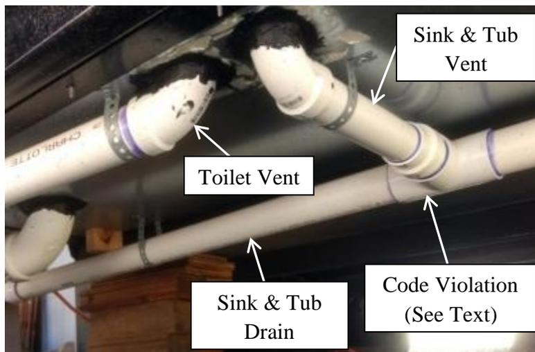
**The DWV system directly below the bathroom vanity shown in the above photo. Note the trailer's structural members (upper left corner of photo in black) that the pipe penetrations avoid.**
