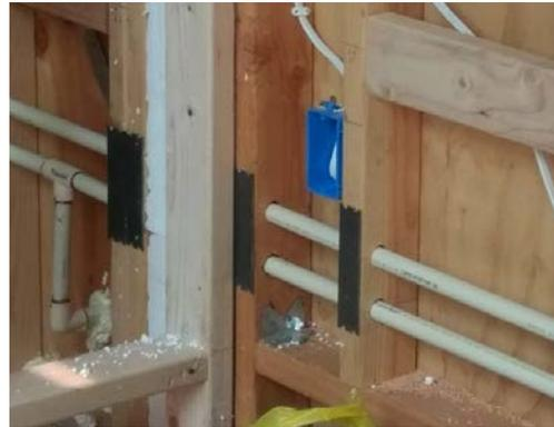
**CPVC piping used in a THOW. The metal nail guards provide protection from accidental puncturing of the pipes when the wall covering is installed.**
