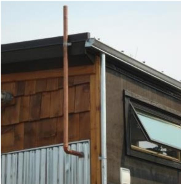
**Left: Copper vent piping through a THOW sidewall. Copper is code approved, but uncommon due to cost.**
