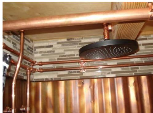
**Copper piping used in a THOW. This is the only THOW I've seen that used copper. The builder used push-to-connect fittings as opposed to soldering joints and fittings.**
