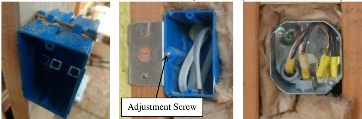
**Left:** A 1-gang, 18 in<sup>3</sup> plastic electric box (Carlon Model #B118A) used for many switches and receptacles.
