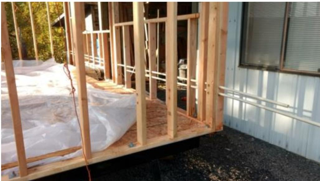
**CPVC water supply piping placed in walls prior to wall sheathing installation. The piping extending past the front of the trailer will be cut and connected to pipes not yet installed in the front wall.**
