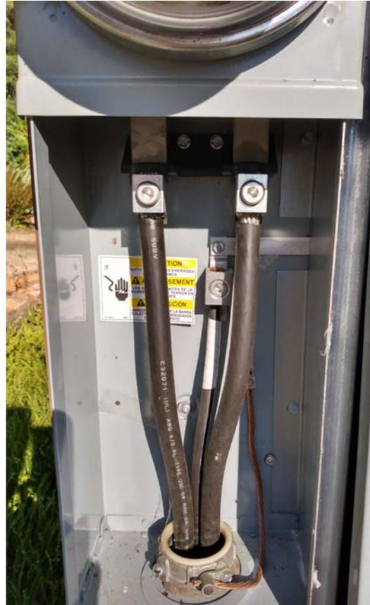
**This photo shows a 3-wire service just prior to the electric meter. Downstream of the meter is a 200 amp main circuit breaker panelboard. The hot wires are 4/0 AWG aluminum.**
