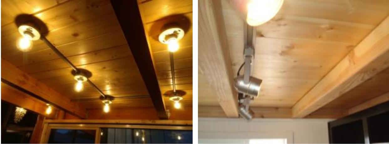
**Left:** Exposed electric boxes and conduit on the underside of a THOW loft floor. The light fixtures are lamp holders without pull chains (Leviton Model # R50-49875-000) with vintage Edison LED G25 light bulbs.
