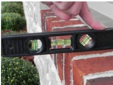
Also, as can be seen in the photo on the right, there is no overhang for the brick sill. The face of the brick sill is flush with the veneer. Consequently, there is no drip edge on the bottom of the cap. The result of this critical error is that any water that manages to run away from the window will drain directly down the exterior face of the masonry wall and pass through
