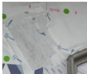
The window flanges are next sealed against the WRB using special sealing tape. The tape is applied to the jambs first (the bottom of the window is not taped) and extends up past the top corner of the window. The drawing on the right shows the proper placement of the lower end of the vertical
