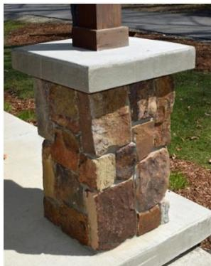
The photo on the left shows an exterior masonry column base with a cast-in-place concrete cap. After the form was built, but before the concrete was placed, a one-half inch diameter half-round piece of wood trim was placed in the bottom of the form to form the drip edge. The photo on the right shows the completed cap from the underneath showing the drip edge. The drip edge is on all four sides of the cap. It is placed just over one-inch away from the face of the stone
