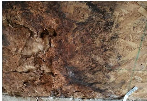
To correct this and all the other construction errors, the entire exterior stone masonry veneer and water resistant barrier were first removed from the building. All plywood sheathing was inspected and the water damaged areas were removed and replaced as were the appropriate windows and doors. A few wood studs were also water damaged to the point that they needed to be removed and replaced necessitating appropriate repairs to affected portions of the interior finishes.
