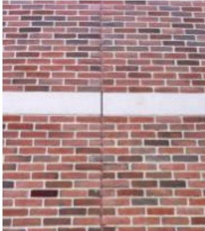
The design of control joints depends on many factors including, but not limited to, fire resistance rating, lateral loads on the wall (including wind, earthquakes, etc.), shrinkage of the materials, amount and types of horizontal reinforcement in the wall, height and thickness of the wall, etc. Also, placement of the control joint in the wall may affect the load distribution. For example, placing a control joint next to a lintel will eliminate arching action from occurring. In such a case, the
