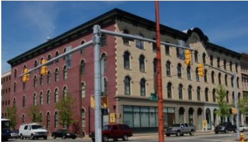
The four story building shown on the left is a good example of using arches as load bearing structural supports. The red clay brick exterior on the left side of the building is a load bearing solid masonry wall with multiple arched openings above the windows. Wooden floor joists bear on the 18-inch thick masonry walls above the arches. My partners and I
