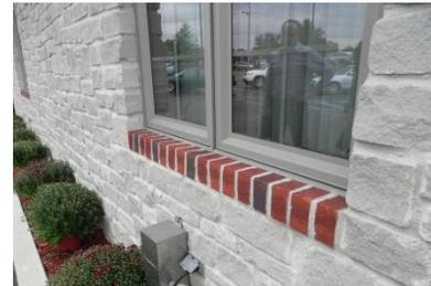
In our discussion of copings and caps in this course, we noted that a window sill is considered a cap on the masonry veneer below the window. The function of the sill is to protect the masonry from water penetration by sealing the top of the wall, providing a slope to drain the water away from the window, and to provide a drip edge to allow the drain water to fall to the ground without necessarily washing over the masonry.
