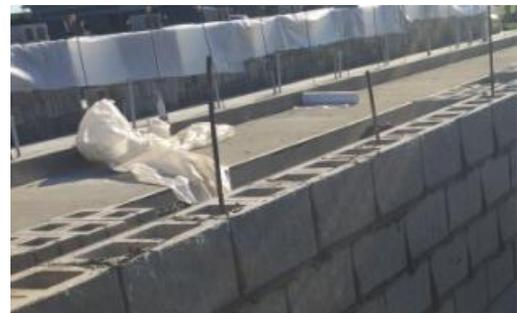
The specifications define two types of grout – fine and coarse. Fine grout contains sand, which is smaller than 3/8 inch in diameter, as its only aggregate. Coarse grout allows pea gravel, which is smaller than 1/2 inch in diameter, in addition to the sand. Mix proportions for grout are shown in the table on the next page. Hydrated lime, which helps in sealing very small cracks, is added
