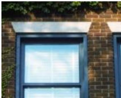
Here are two more examples of masonry arches above windows. The photo on the left seems to just be a simple lintel. In fact, because its supports do not bear directly downward on supporting masonry, but rather “push out” on the wall, it is considered a Flat or Jack arch.
