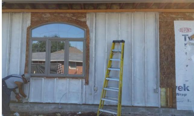
In addition to the poor quality workmanship, there were design errors. The plans prepared for the construction of the building were poorly done and incomplete. For example, the plans had no flashing details for openings in the walls, and no detail for the proper installation of the rowlock brick window sills. And, finally, there was no competent inspector working for the owner to oversee the construction to help guard against such mistakes.
