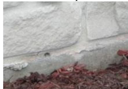
The expert's report cited several specific issues with the construction of the masonry veneer, including several instances of improper flashing installation, no proper weep holes, improper
