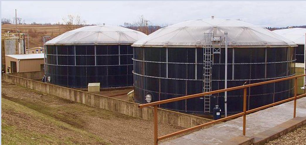
Figure 8: Two 400,000 gallon equalization tanks for landfill leachate pretreatment.
