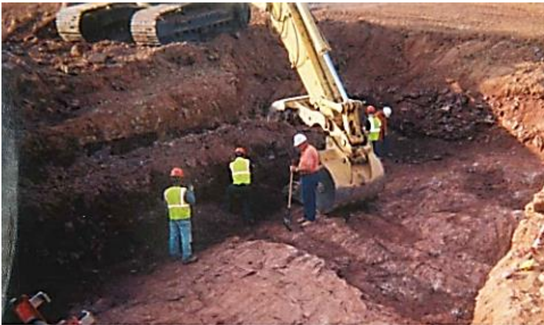
Shale Excavation for Bridge Footing
